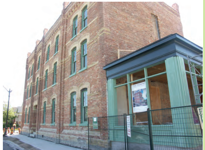
West side of The Tremont with the cafe and terrace
