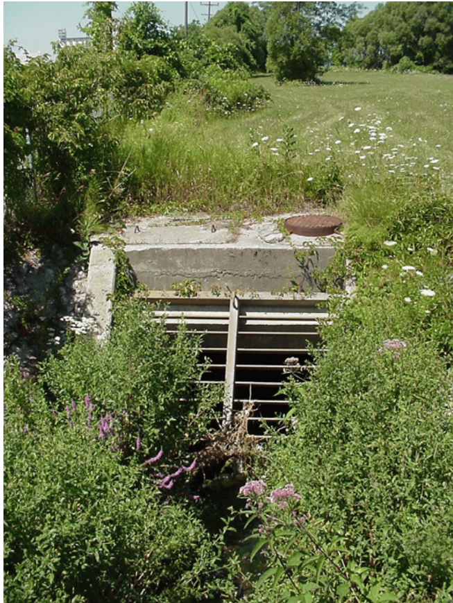
Plate 10: Stormwater tunnel located beneath the grassy area.
