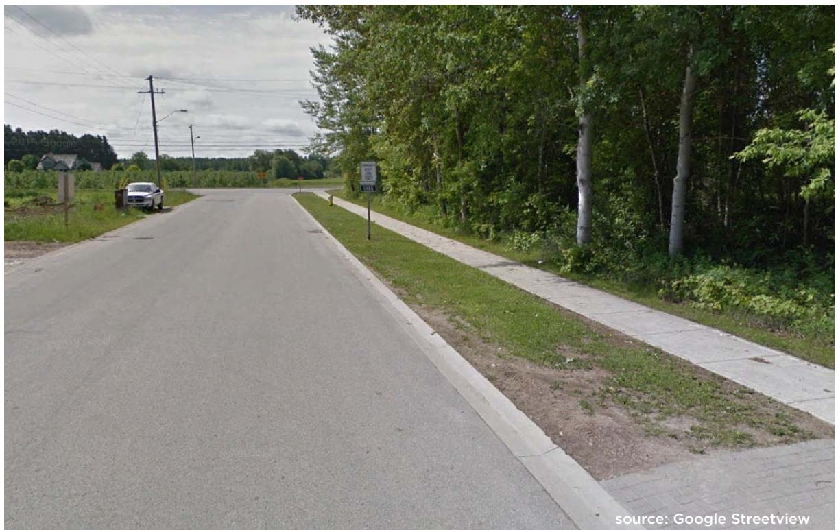
Looking south along Saunders Street from proposed south access point
