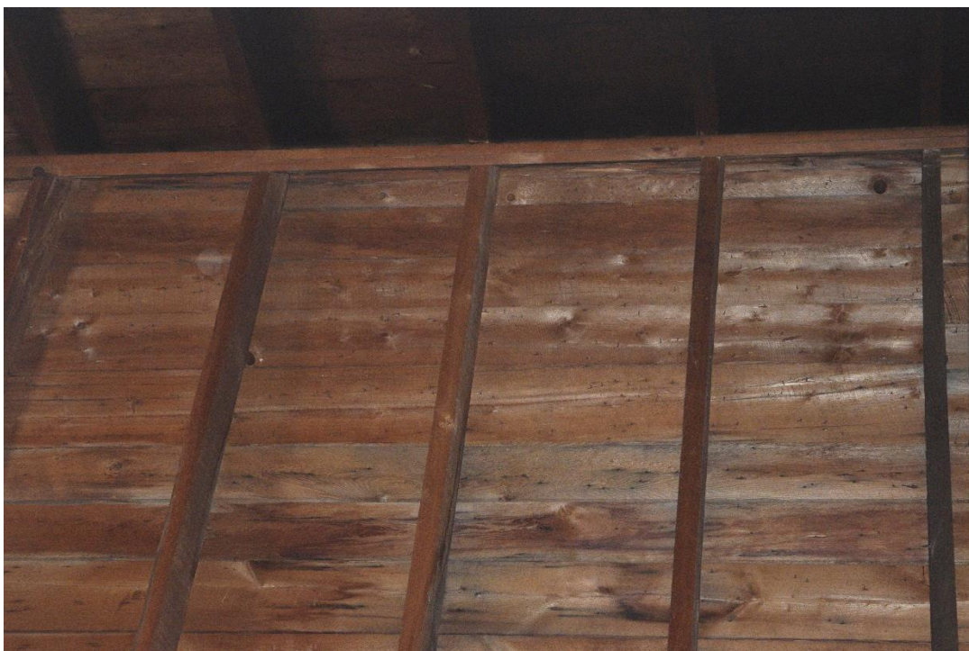
Figure 68: Room framing and planking as seen through the attic access (May 2016).
