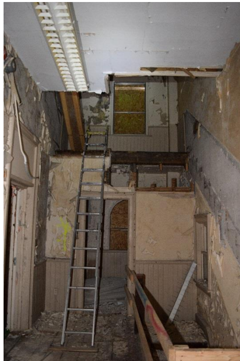
Figure 49: First level of the north transept, facing west (May 2016).
