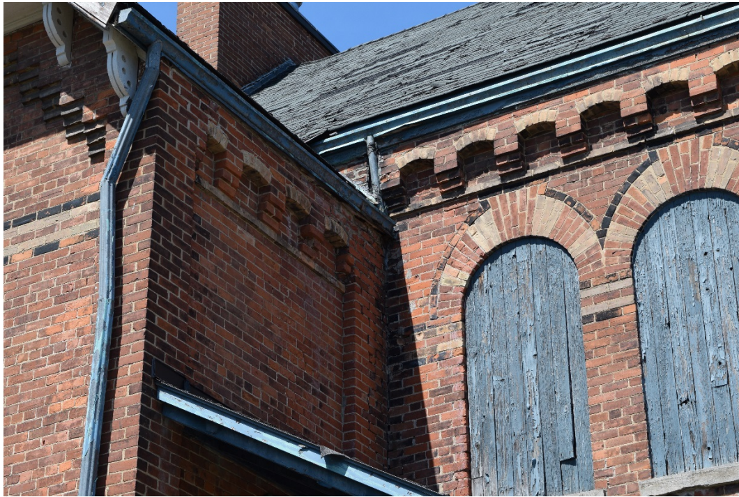
Figure 37: Arched corbel table on the east wall of the south transept (left) and south wall of the main block (right) (May 2016).
