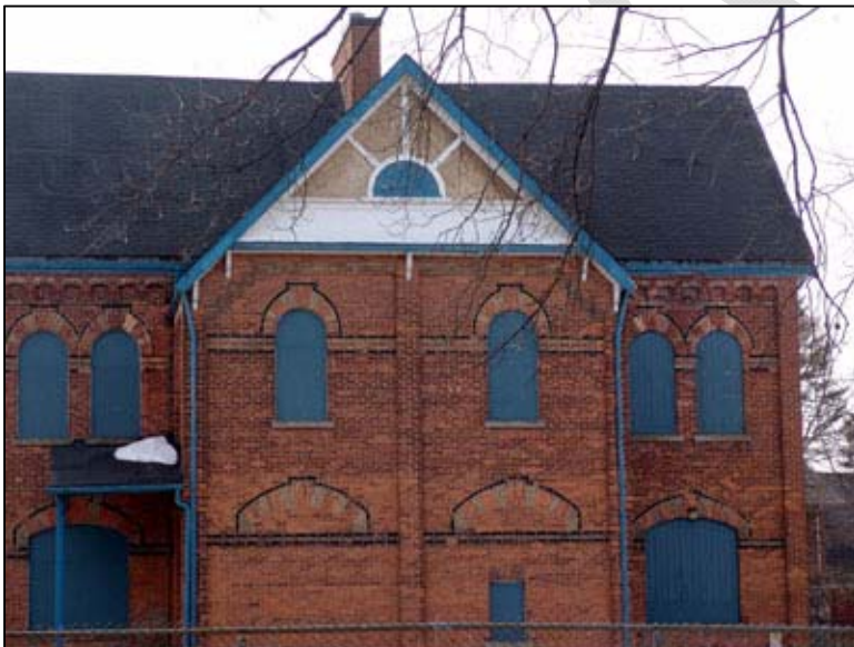
Figure 10: North façade, March 15, 2007. Detail of segmental (lower level) and round (upper) window openings, step-like brick corbelling within the gable, sunburst gable design, wood brackets, brick arcading at the eaves, and use of red/cream/black bricks.
