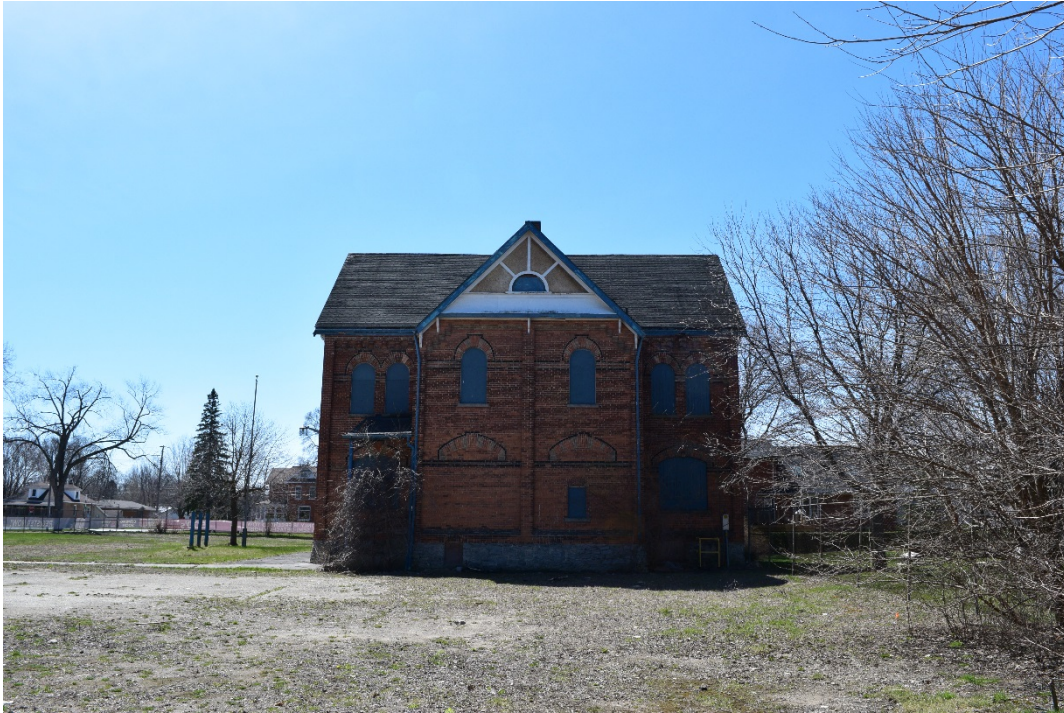
Figure 11: View of the Study Area facing south showing east and north lawns and north façade of the Annex (April 2016).
