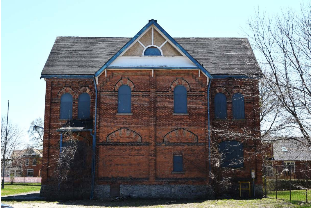
Figure 27: The north façade of the Annex (May 2016).
