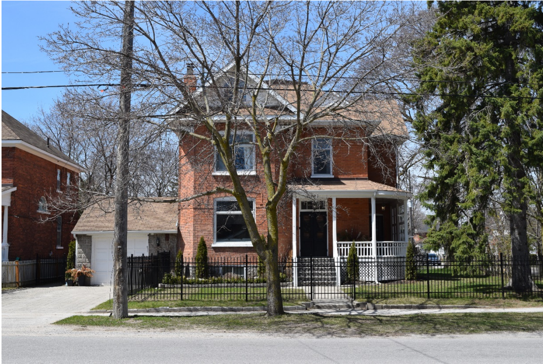
Figure 19: View facing west of the municipally designated heritage property at 402 Maple Street (April 2016).
