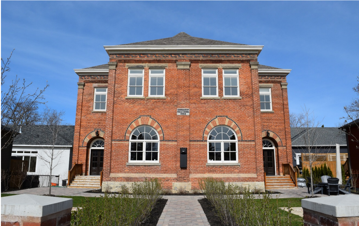
Figure 74: The rehabilitated and adaptively re-used East Ward/ Connaught School at 125 Napier Street in the Town of Collingwood (April 2016).
