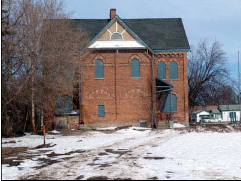
Figure 17: South façade, March 15, 2007.
