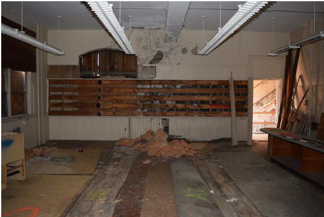
Figure 53: View facing south of the east first-level classroom (May 2016).
