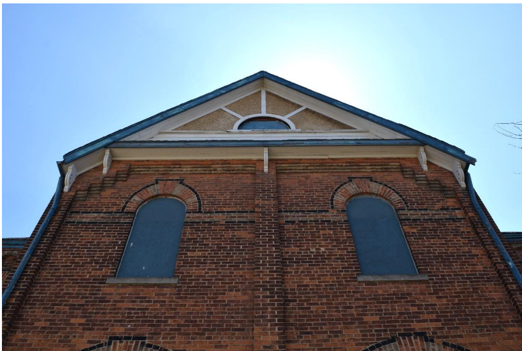
Figure 33: Lesenes or pilaster strips on the corners and centre of the north transept (May 2016).
