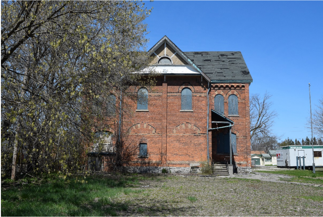
Figure 31: The south façade of the Annex (May 2016).
