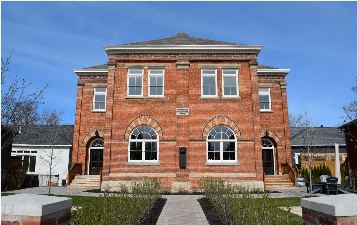
Figure 73: The rehabilitated and adaptively re-used East Ward/ Connaught School at 125 Napier Street in the Town of Collingwood (April 2016).
