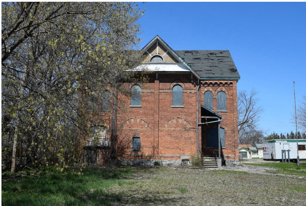
Figure 30: The south façade of the Annex (May 2016).
