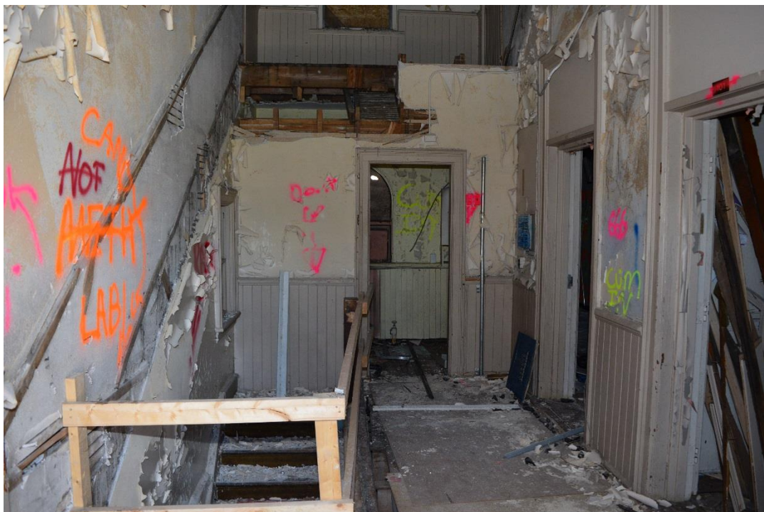
Figure 50: First level of the south transept, facing west (May 2016).
