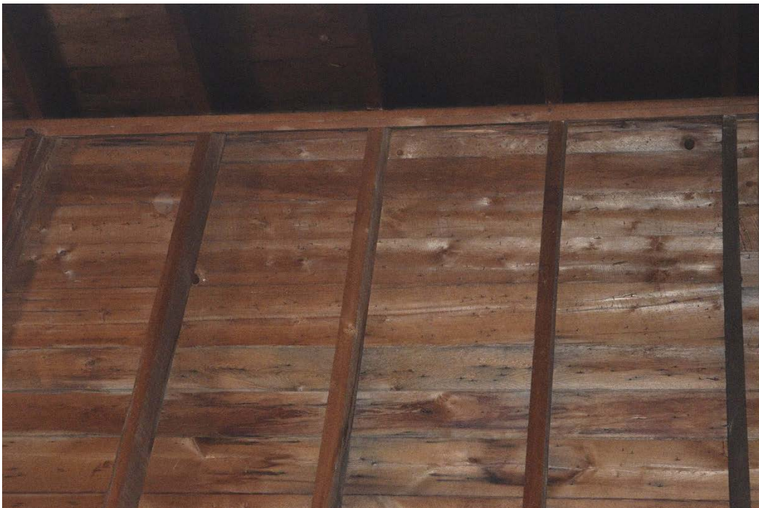
Figure 69: Room framing and planking as seen through the attic access (May 2016).
