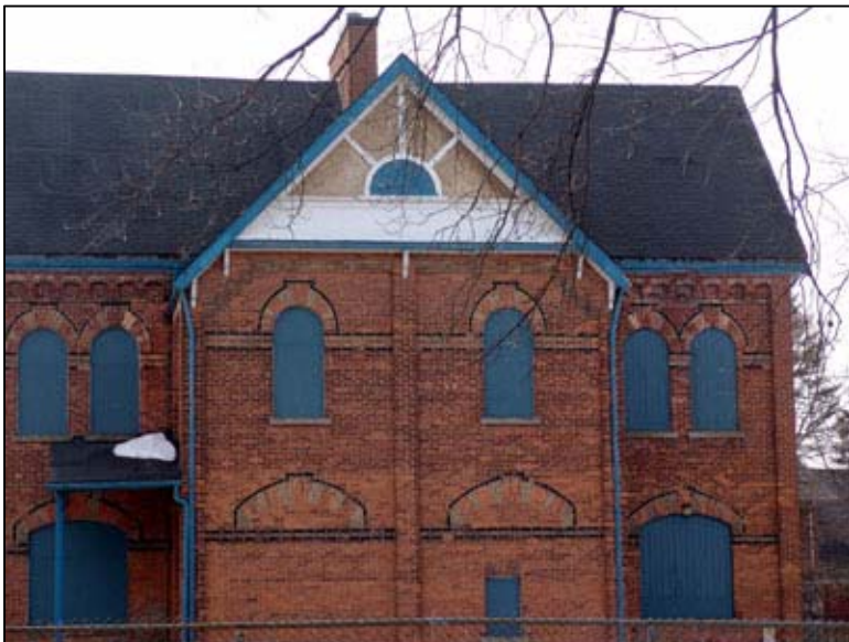
Figure 10: North façade, March 15, 2007. Detail of segmental (lower level) and round (upper) window openings, step-like brick corbelling within the gable, sunburst gable design, wood brackets, brick arcading at the eaves, and use of red/cream/black bricks.
