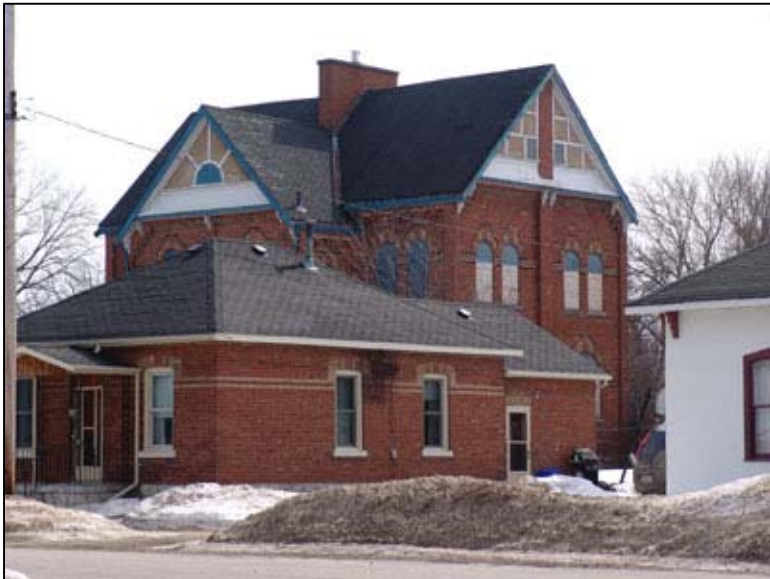
Figure 18: West façade (R), north façade (L), March 15, 2007. The brick dwelling abuts the northwest corner of the property.
