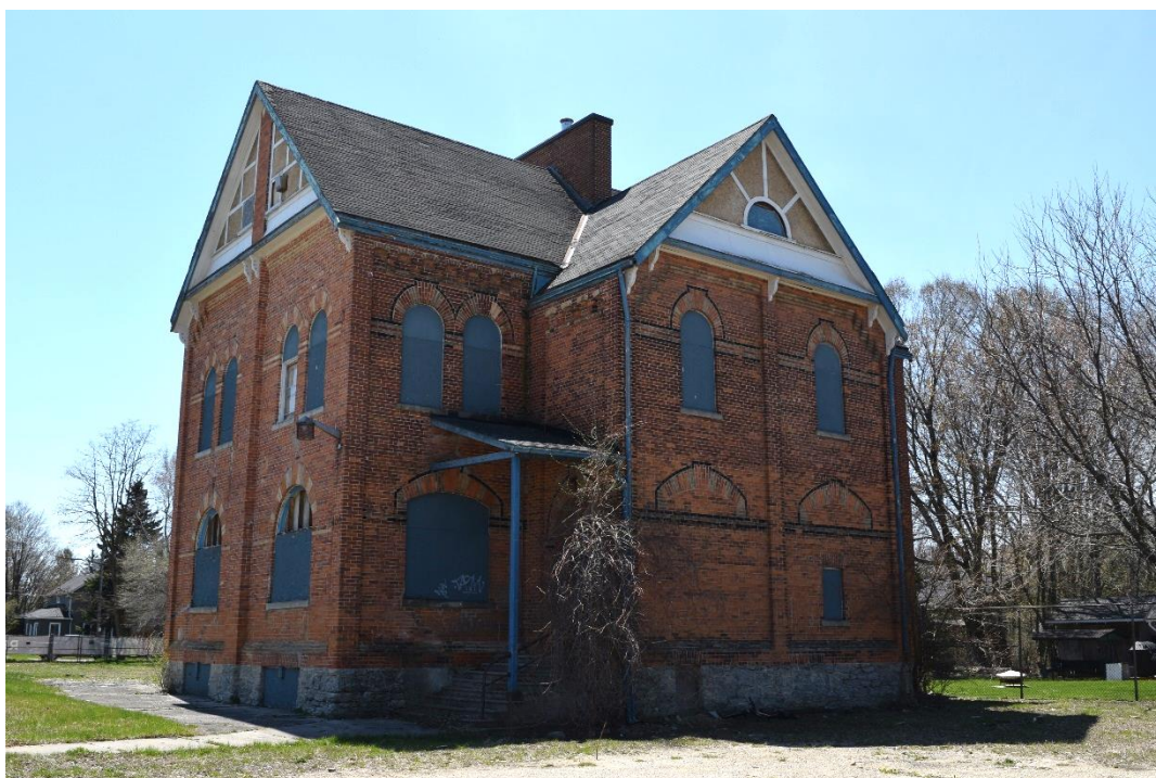
Figure 27: The east and north façades of the Annex (May 2016).
