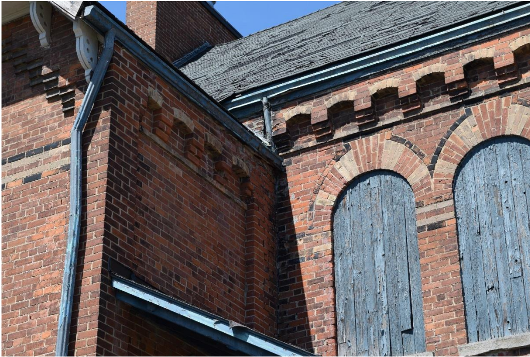
Figure 36: Arched corbel table on the east wall of the south transept (left) and south wall of the main block (right) (May 2016).
