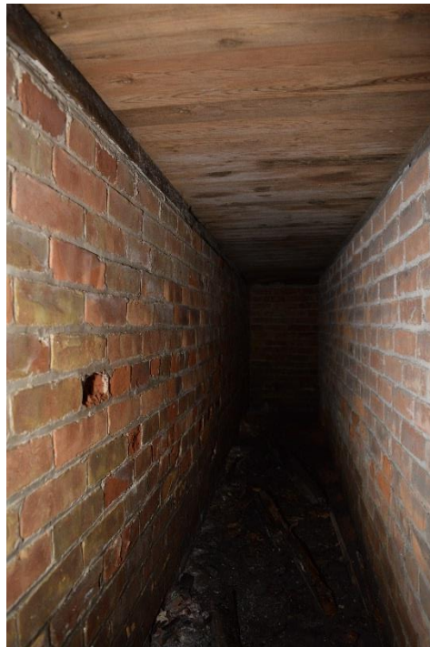
Figure 45: Interior of the brick channel running west from the furnace (May 2016).
