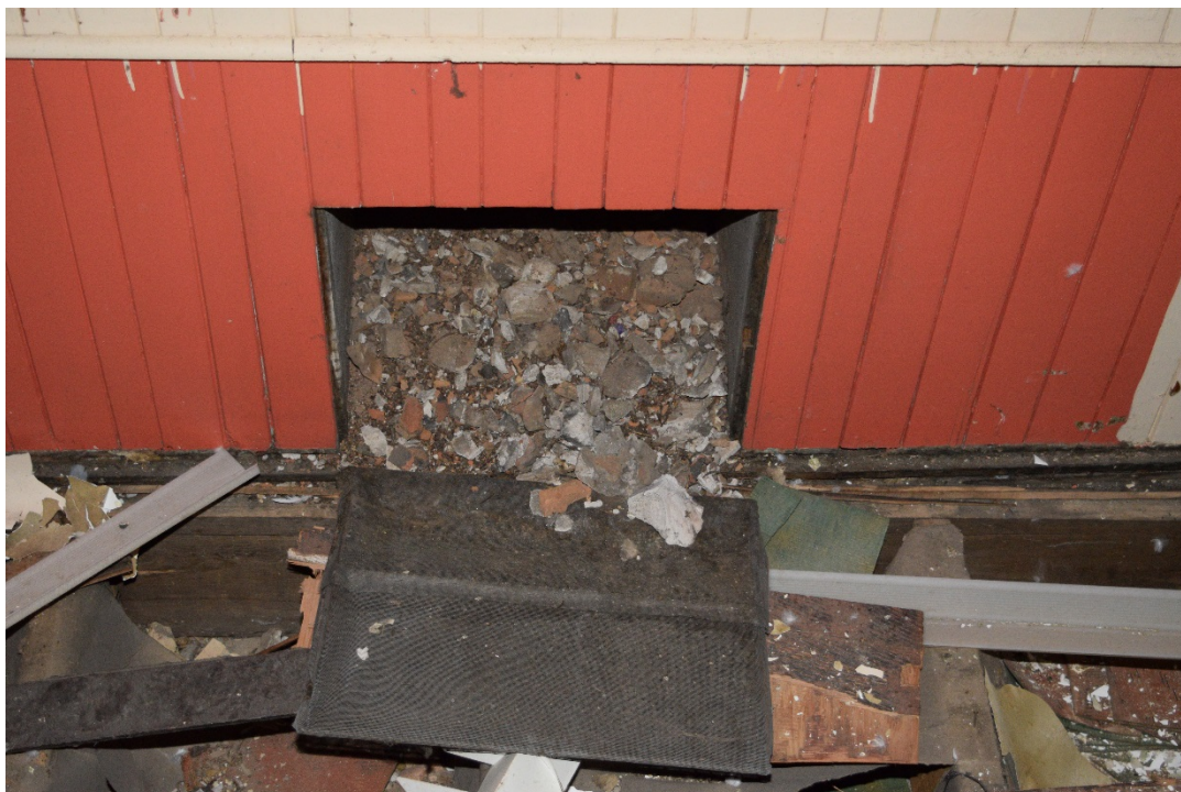
Figure 67: Coal chute in the second level classroom (May 2016).
