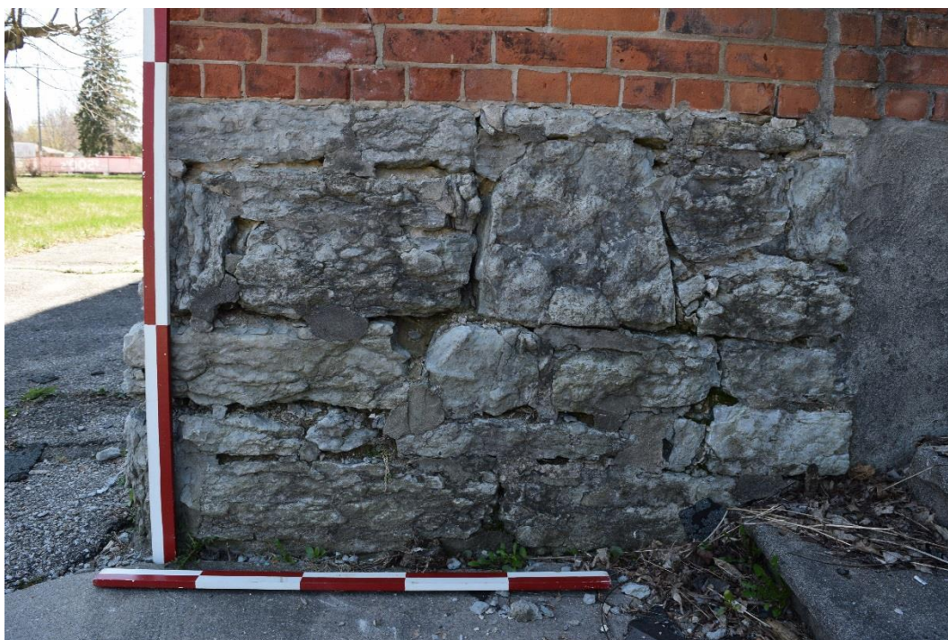
Figure 31: The coursed rubble foundation (northeast corner of the main block) (May 2016).
