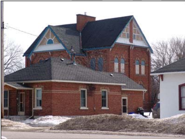
Figure 18: West façade (R), north façade (L), March 15, 2007. The brick dwelling abuts the northwest corner of the property.
