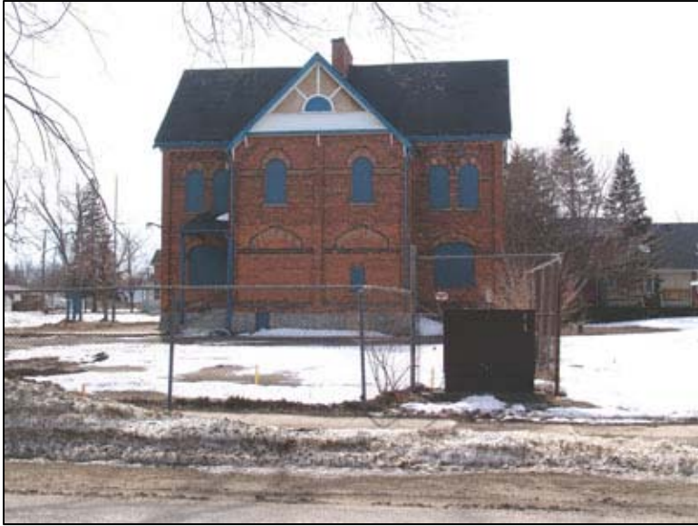
Figure 9: North façade of Annex, March 15, 2007.
