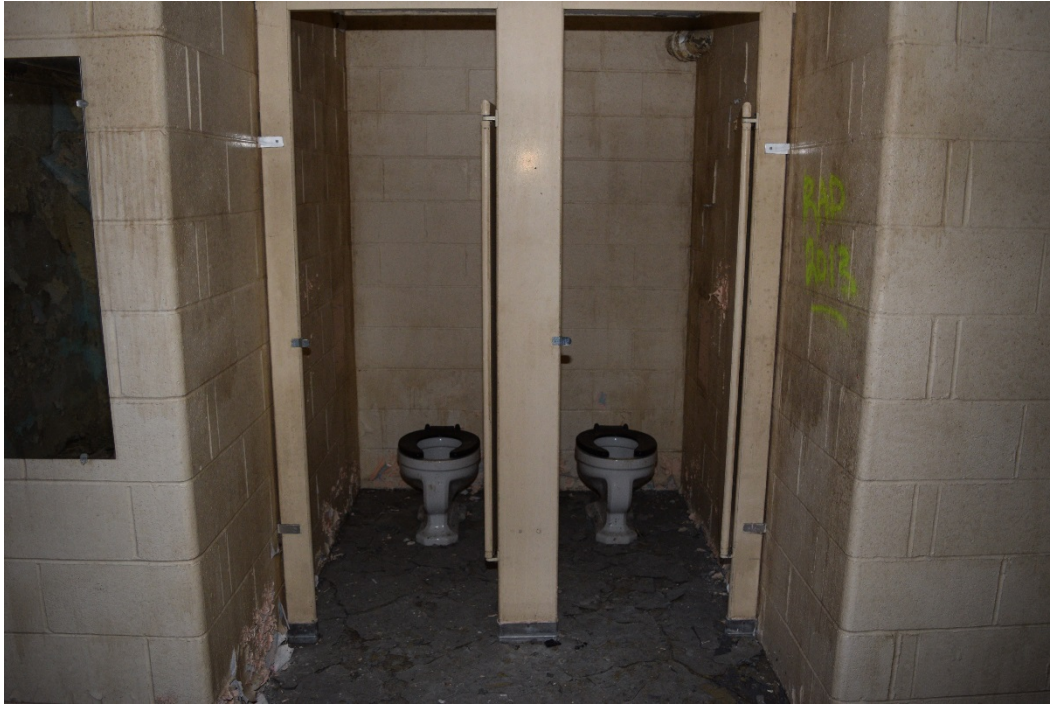
Figure 48: Toilet stalls in the 'Boys' bathroom (May 2016).
