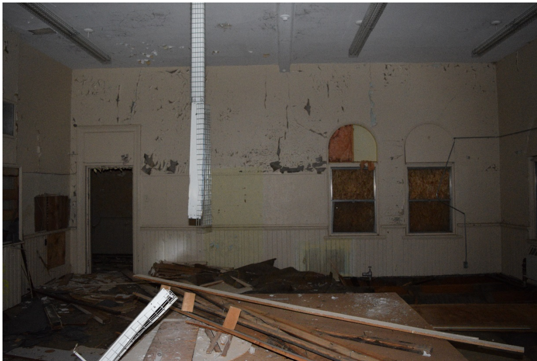
Figure 64: View facing north of the east second-level classroom (May 2016).
