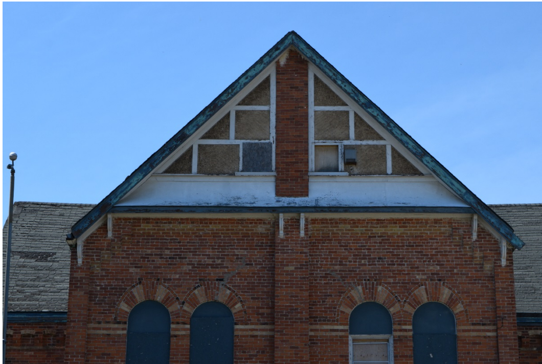
Figure 39: 'Stick' decoration on the east gable of the main block (May 2016).
