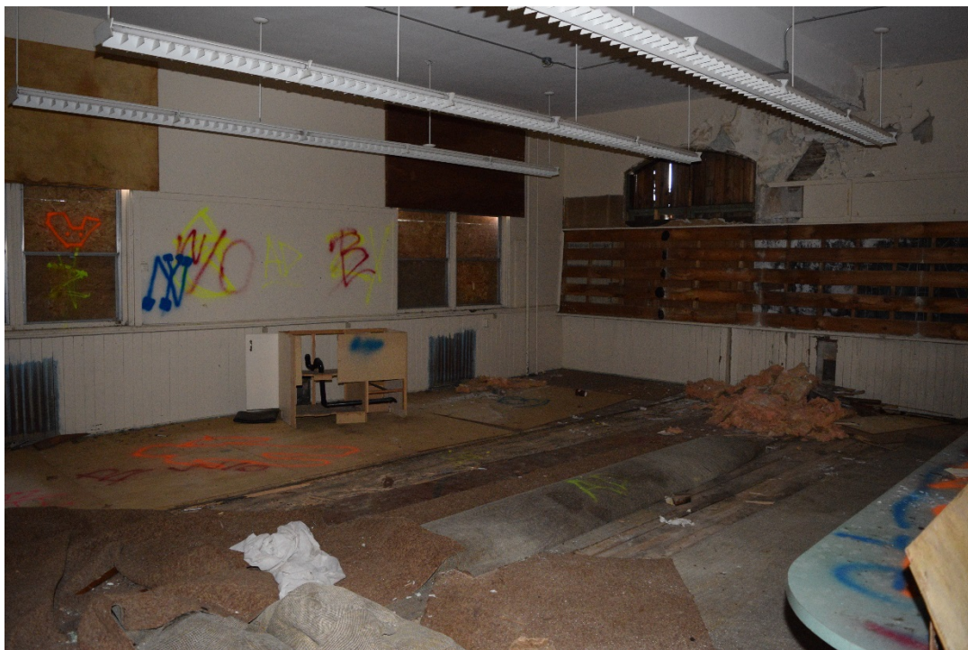
Figure 53: View facing southeast of the east, first-level classroom (May 2016).
