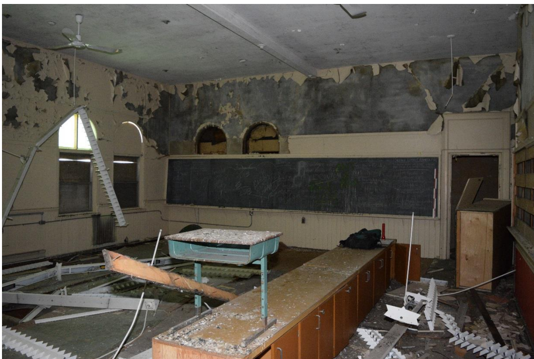
Figure 62: View facing south of the west second-level classroom (May 2016).
