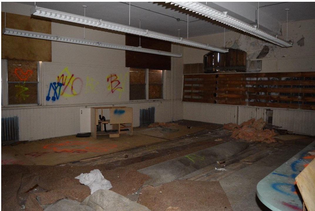
Figure 52: View facing southeast of the east, first-level classroom (May 2016).
