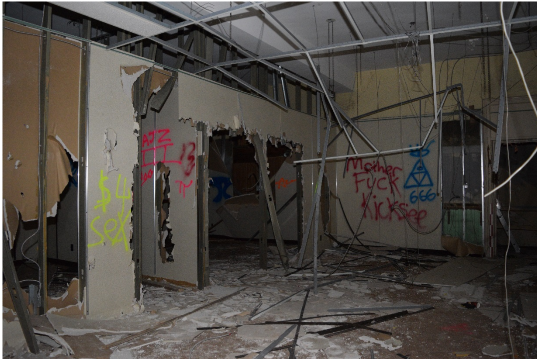
Figure 56: View facing north of the west classroom offices (May 2016).
