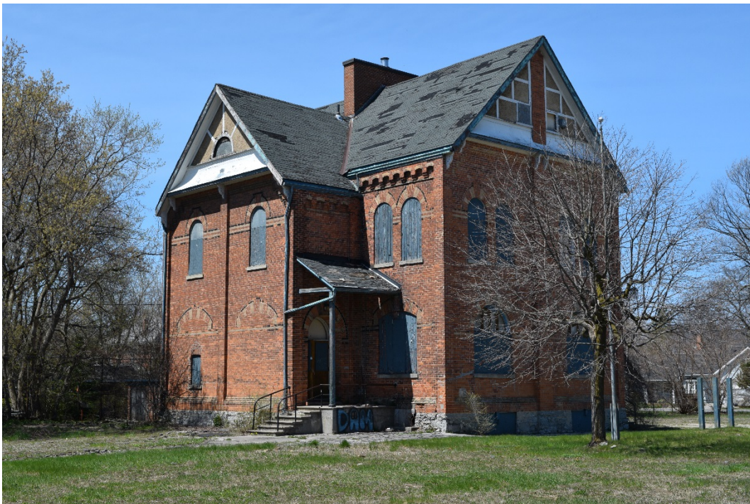
Figure 30: The south and east façades of the Annex (May 2016).
