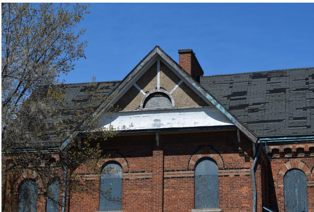
Figure 39: 'Sunburst' Stick decoration and pent roof on the south transept cross-gable (May 2016).
