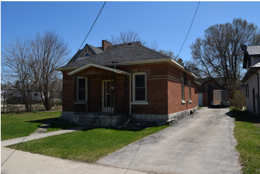
Figure 24: View facing southeast of a heritage structure on Fifth Street northwest of the Annex (which can be seen in the background) (May 2016).
