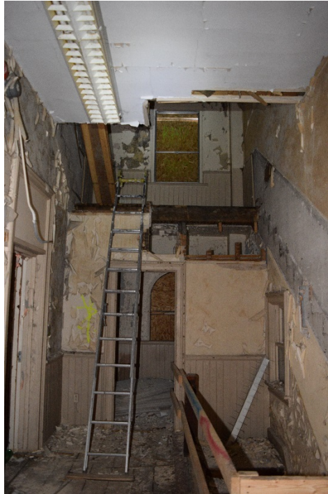
Figure 50: First level of the north transept, facing west (May 2016).
