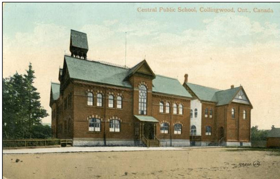
Figure 5: North façade of Central School and Annex circa 1905 (from Murdoch 2015:16, orig. Collingwood Museum X969-152-1).
