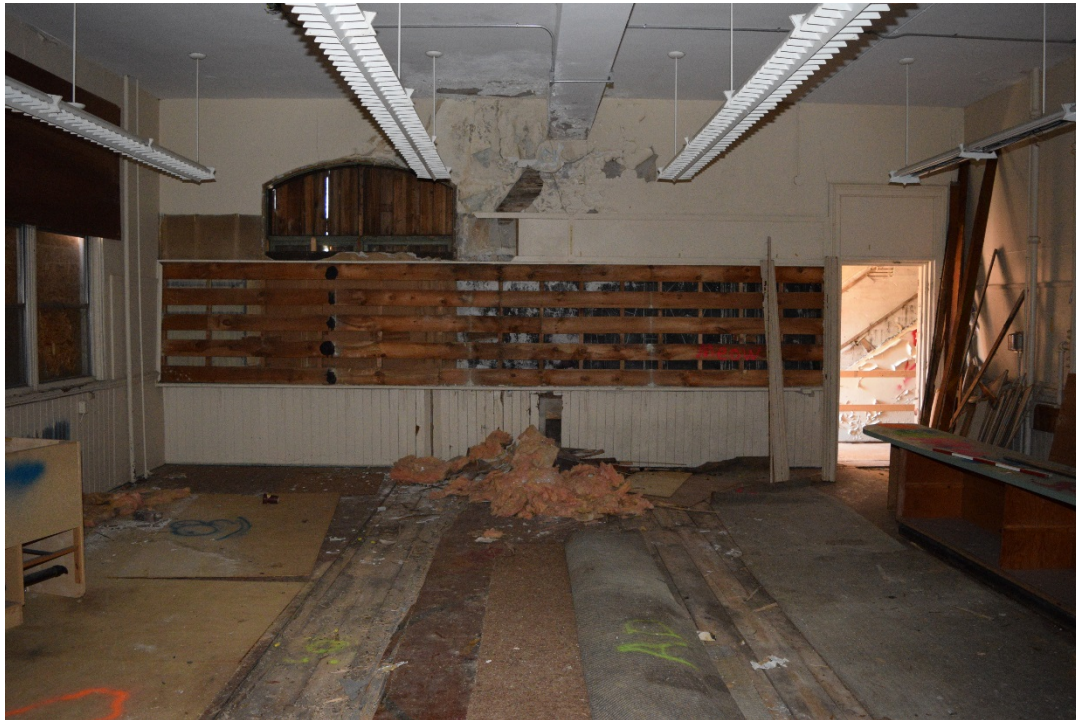
Figure 54: View facing south of the east first-level classroom (May 2016).
