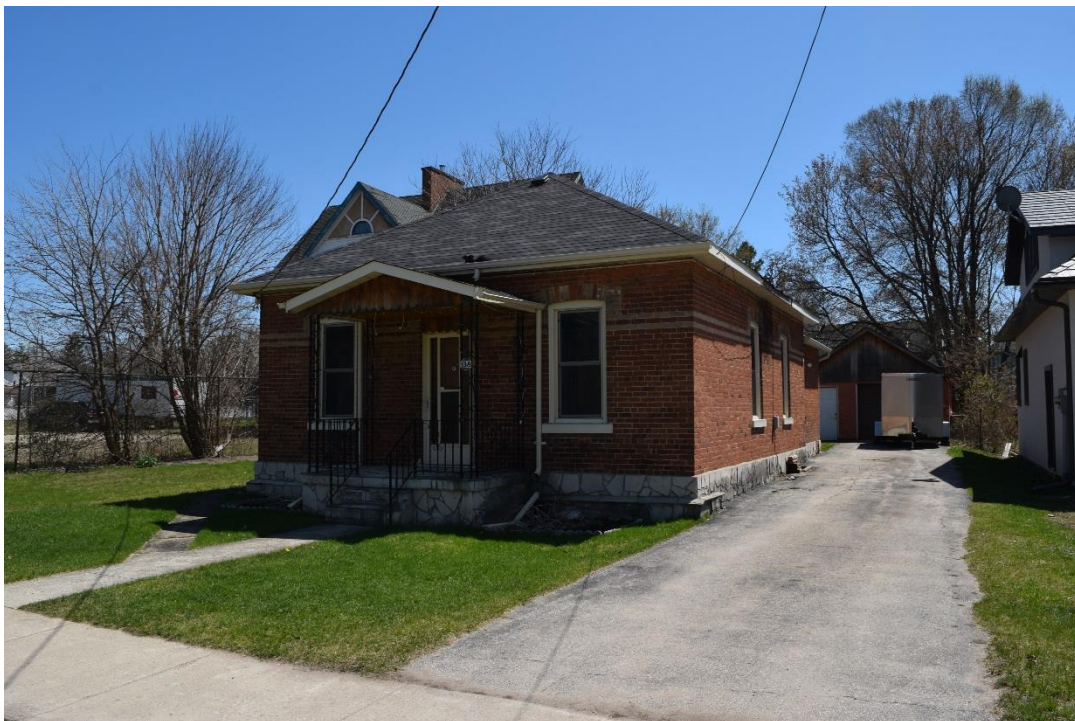
Figure 23: View facing southeast of a heritage structure on Fifth Street northwest of the Annex (which can be seen in the background) (May 2016).
