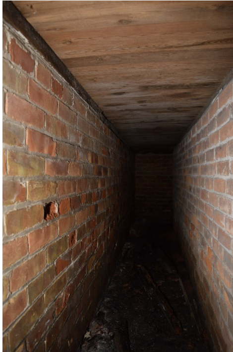
Figure 46: Interior of the brick channel running west from the furnace (May 2016).
