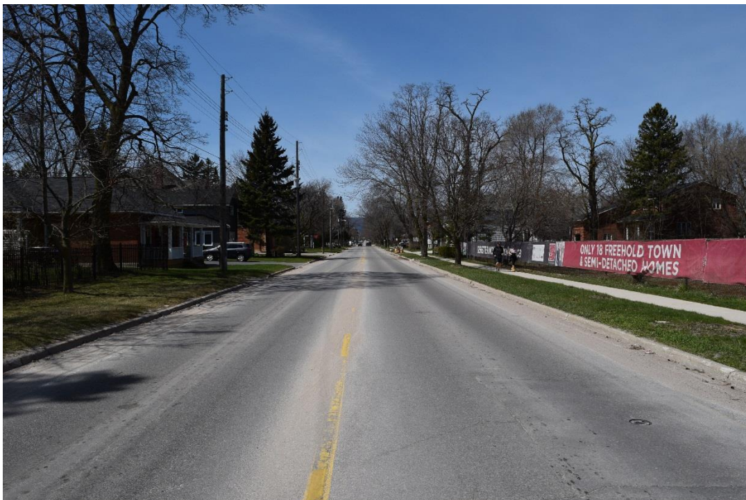
Figure 25: Streetscape of Sixth Street facing west from near the intersection with Maple Street (April 2016).
