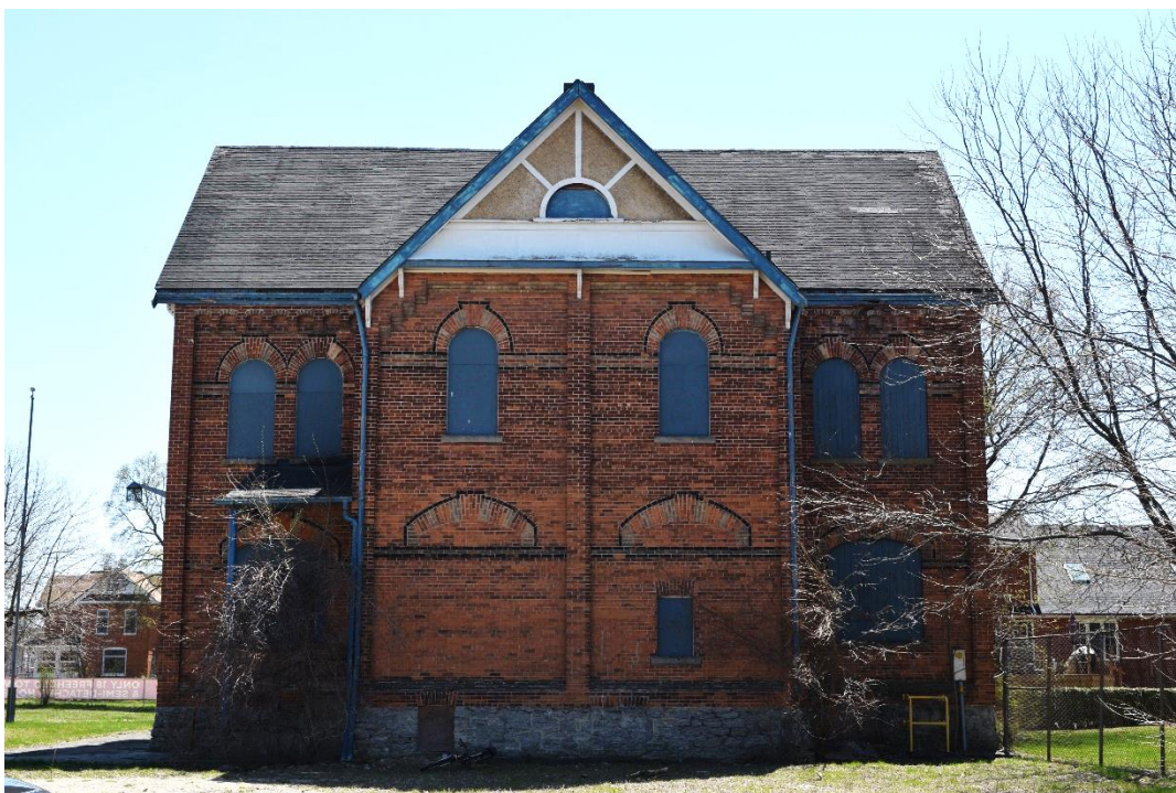
Figure 26: The north façade of the Annex (May 2016).
