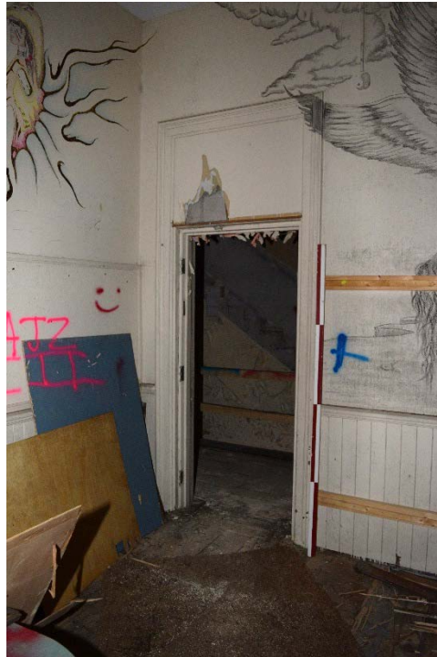
Figure 58: Door architrave and transom in the east first-level classroom (May 2016).
