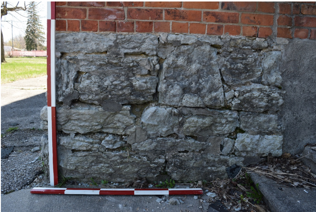
Figure 32: The coursed rubble foundation (northeast corner of the main block) (May 2016).
