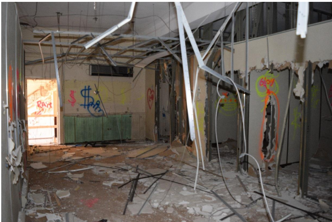
Figure 54: View facing south of the west first-level classroom, now divided into offices (May 2016).
