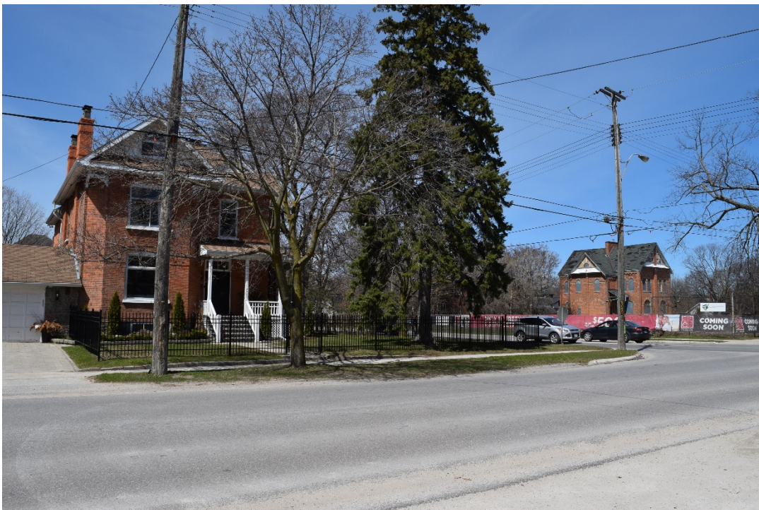
Figure 20: View facing northwest showing the visual relationship between 402 Maple and the Annex (April 2016).
