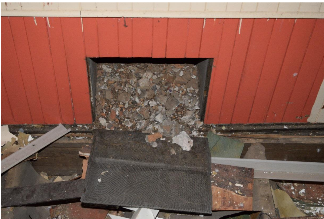
Figure 66: Coal chute in the second level classroom (May 2016).
