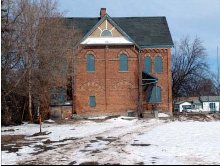
Figure 17: South façade, March 15, 2007.
