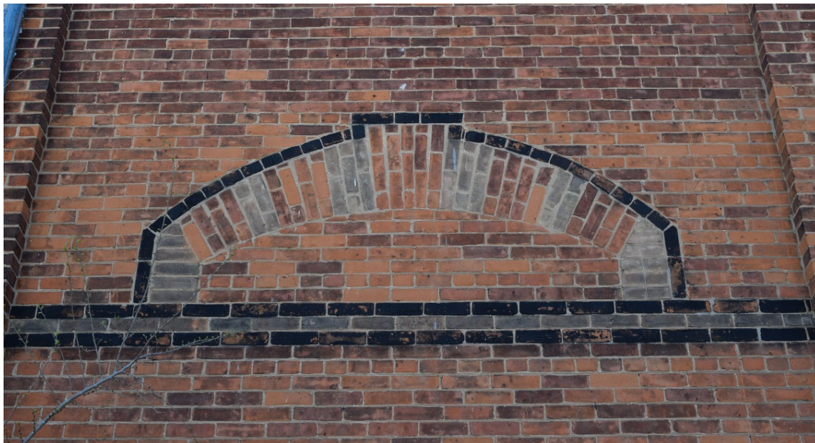
Figure 36: Dichromatic brick belt course and blind window voussoirs on the north wall of the north transept (May 2016).
