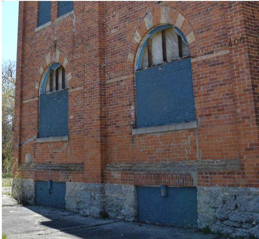
Figure 35: Diocletian windows on the east end wall of the main block (May 2016).
