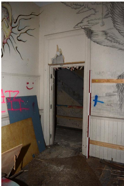
Figure 57: Door architrave and transom in the east first-level classroom (May 2016).
