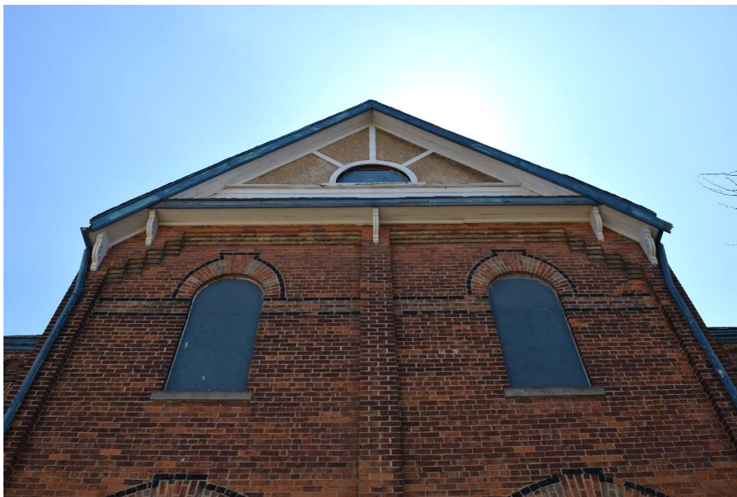
Figure 34: Lesenes or pilaster strips on the corners and centre of the north transept (May 2016).
