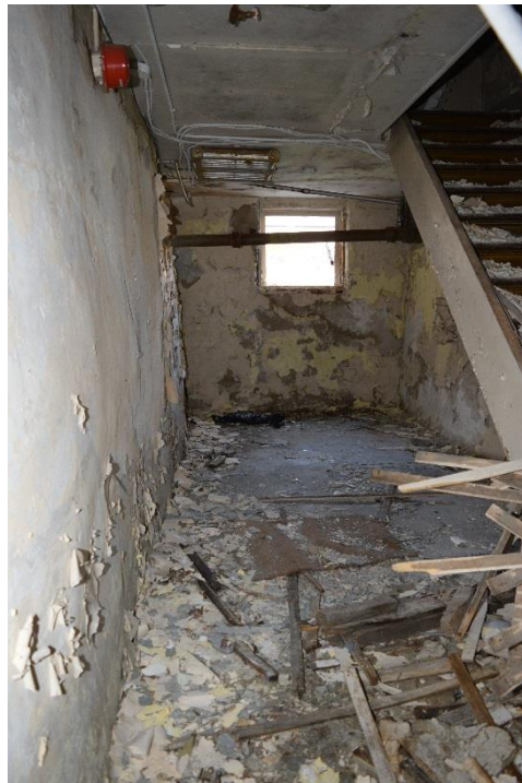
Figure 41: Basement of the north transept, facing west (May 2016).
