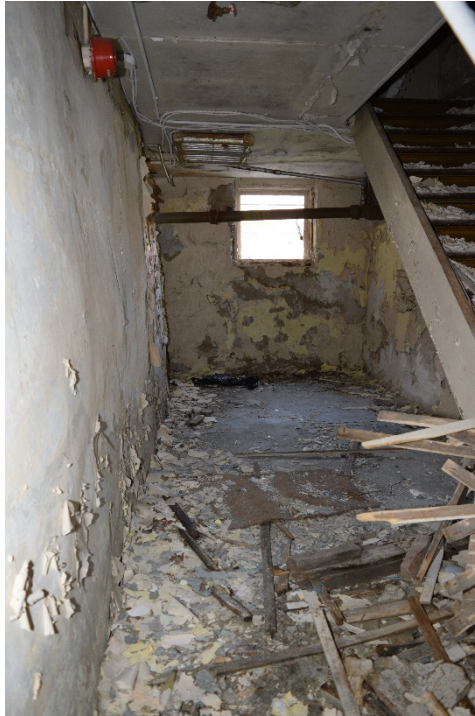
Figure 42: Basement of the north transept, facing west (May 2016).
