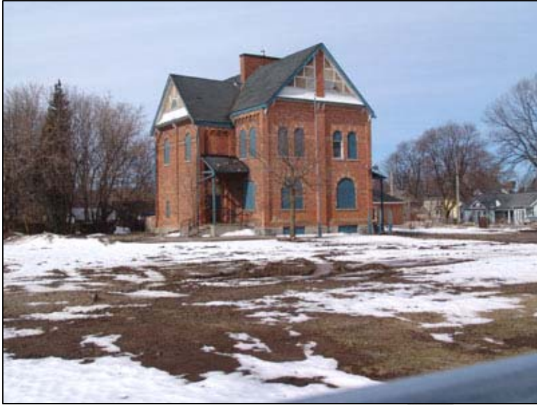
Figure 14: Left: East façade (R), south façade (L), March 15, 2007.
