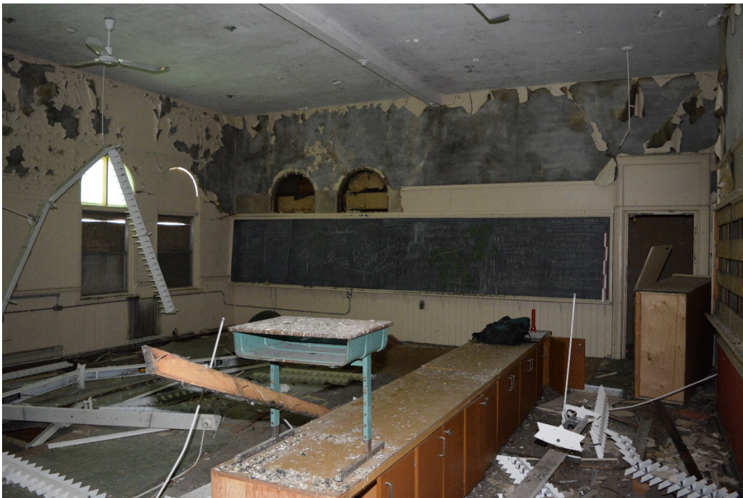
Figure 63: View facing south of the west second-level classroom (May 2016).
