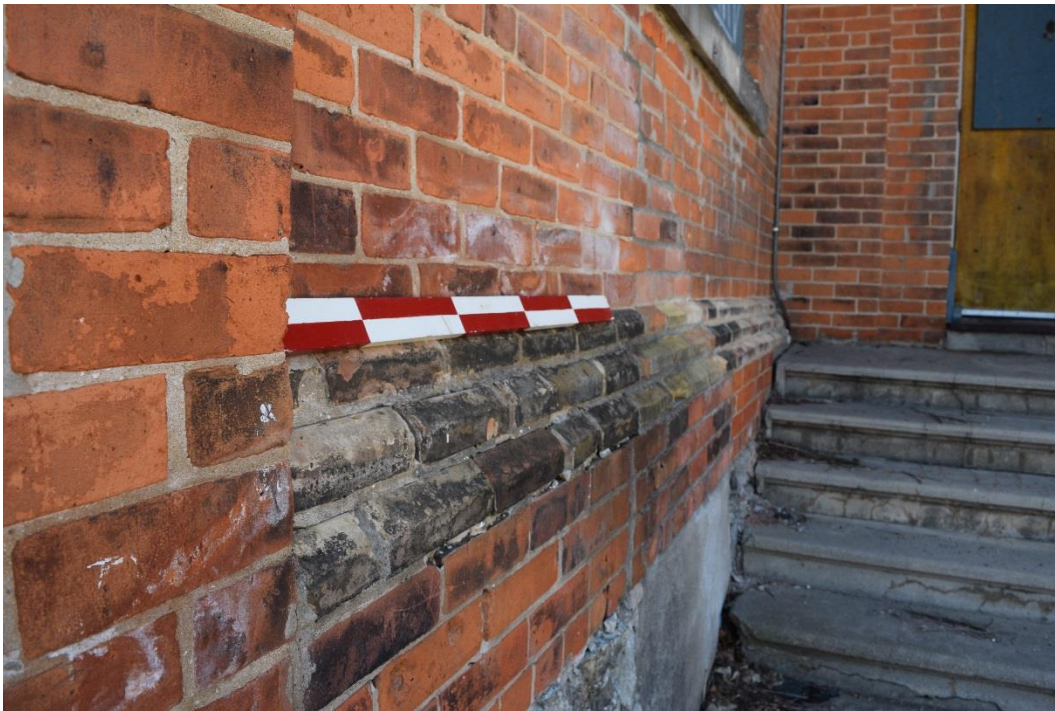
Figure 32: The brick water table (northeast wall of the main block) (May 2016).
