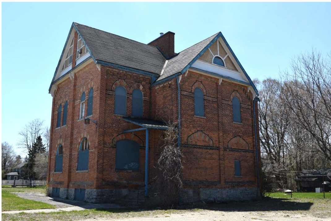
Figure 28: The east and north façades of the Annex (May 2016).
