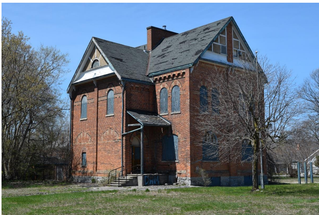
Figure 29: The south and east façades of the Annex (May 2016).
