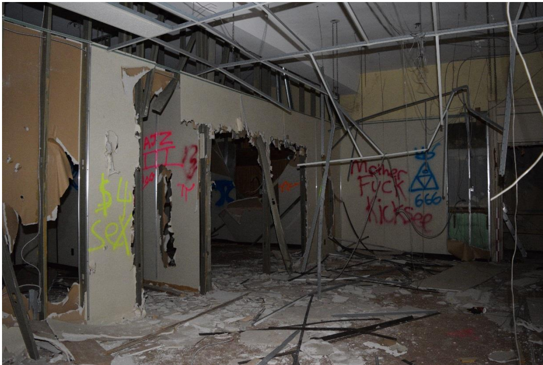
Figure 55: View facing north of the west classroom offices (May 2016).
