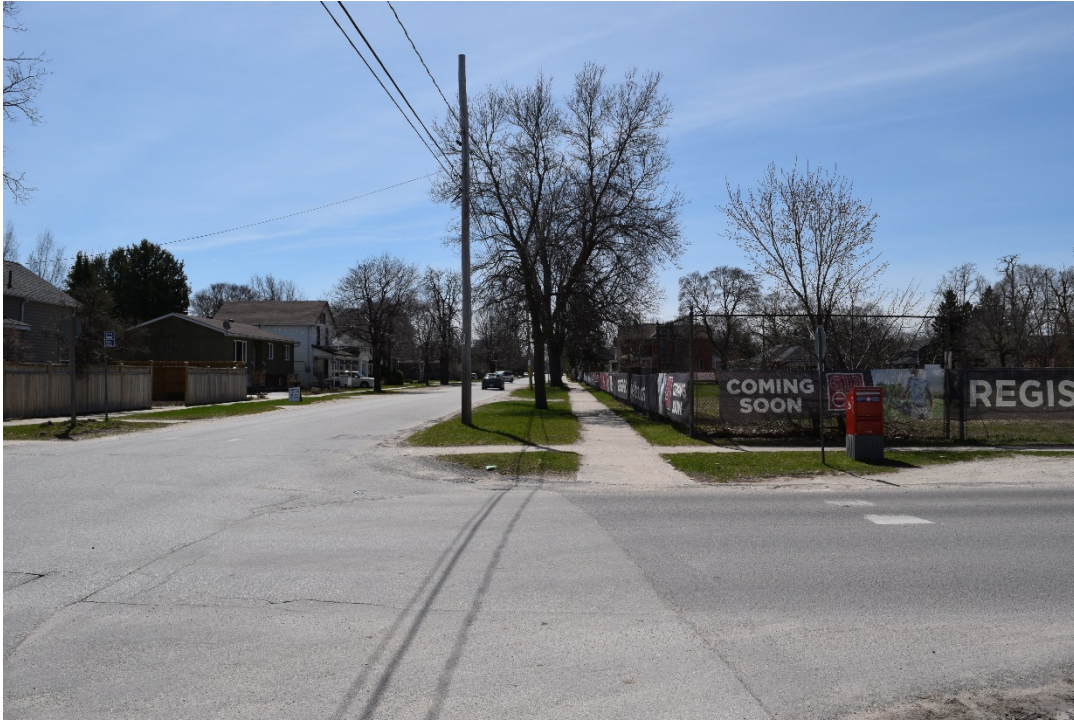
Figure 25: Streetscape of Maple Street facing south from north of Fifth Streets (April 2016).
