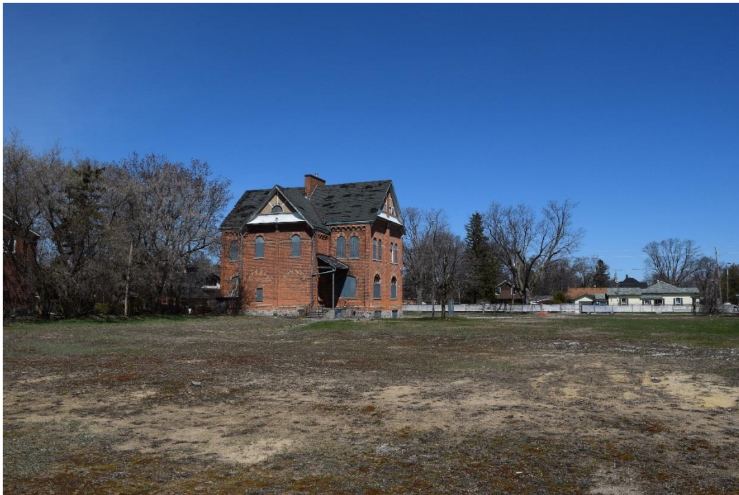
Figure 14: View from the property facing north (April 2016).
