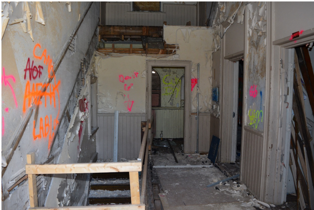
Figure 51: First level of the south transept, facing west (May 2016).
