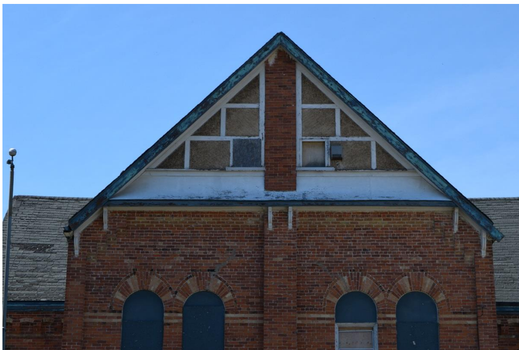
Figure 38: 'Stick' decoration on the east gable of the main block (May 2016).
