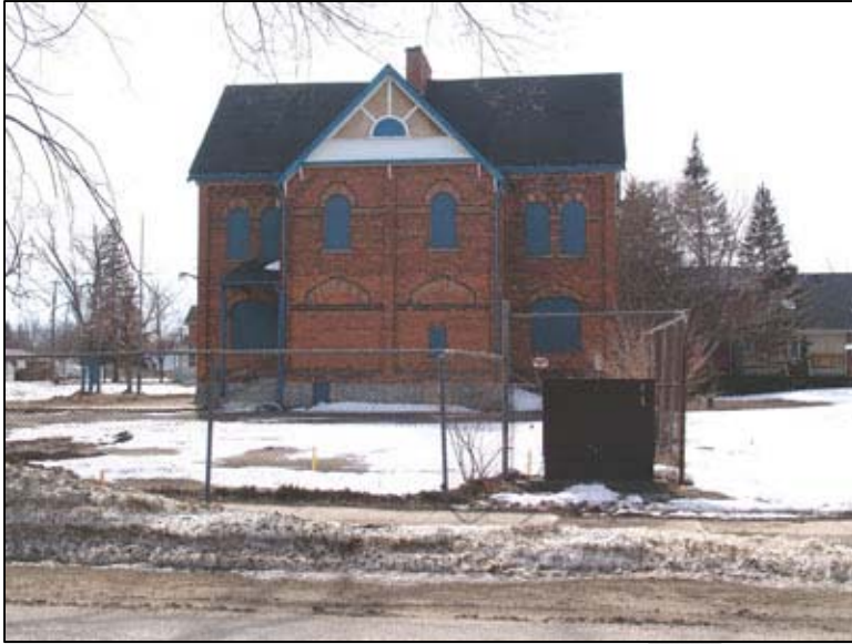
Figure 9: North façade of Annex, March 15, 2007.
