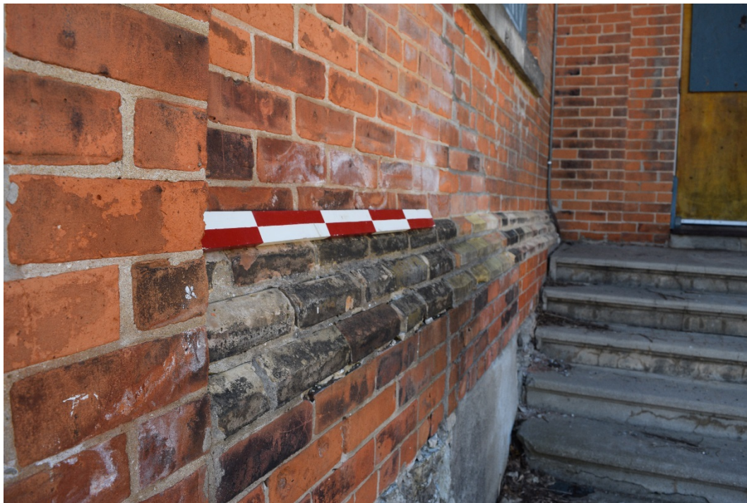
Figure 33: The brick water table (northeast wall of the main block) (May 2016).
