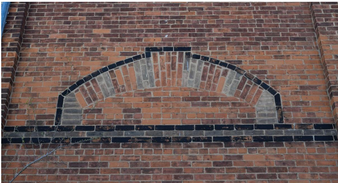
Figure 35: Dichromatic brick belt course and blind window voussoirs on the north wall of the north transept (May 2016).
