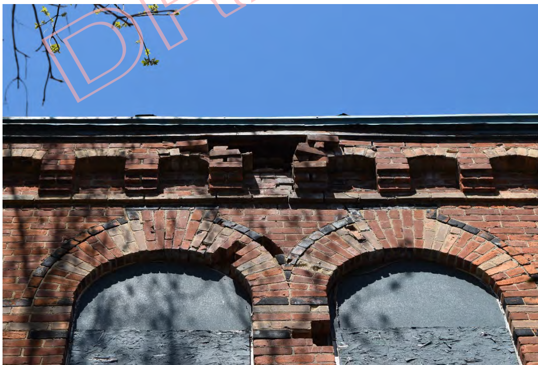
Figure 72: Missing and displaced section of arched corbel table, voussoir, and window column on the southwest façade of the main block (May 2016).
