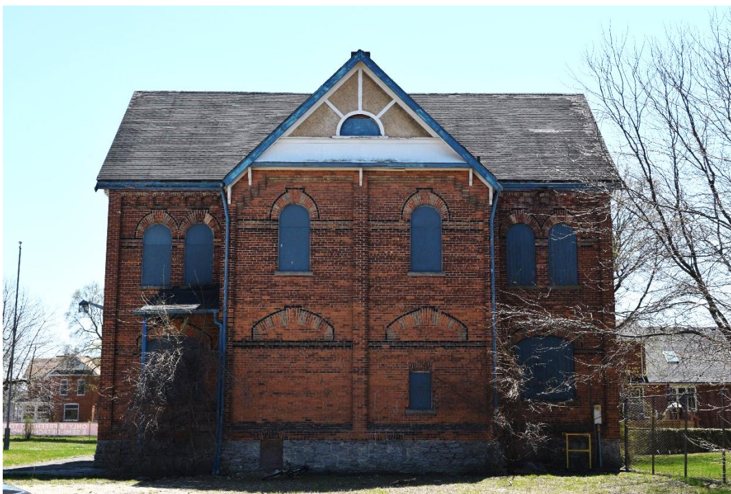
Figure 26: The north façade of the Annex (May 2016).
