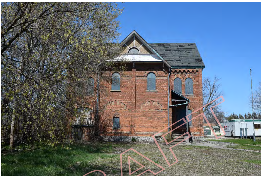
Figure 31: The south façade of the Annex (May 2016).
