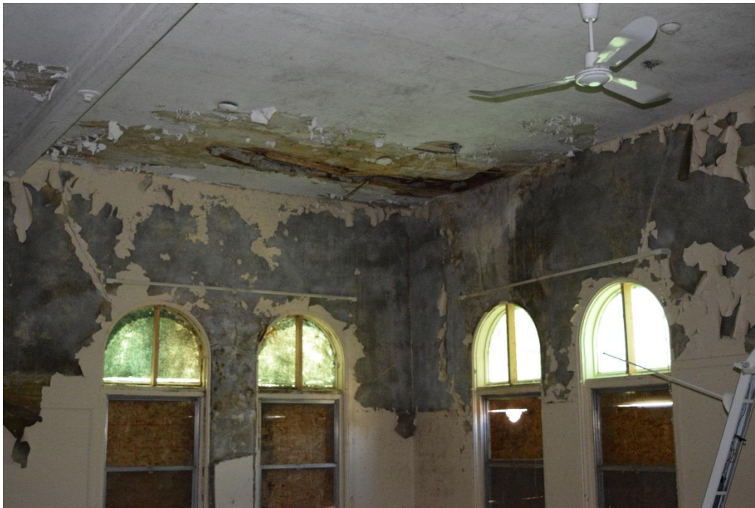
Figure 69: Water damage in the northwest corner of the west second-level classroom (May 2016).
