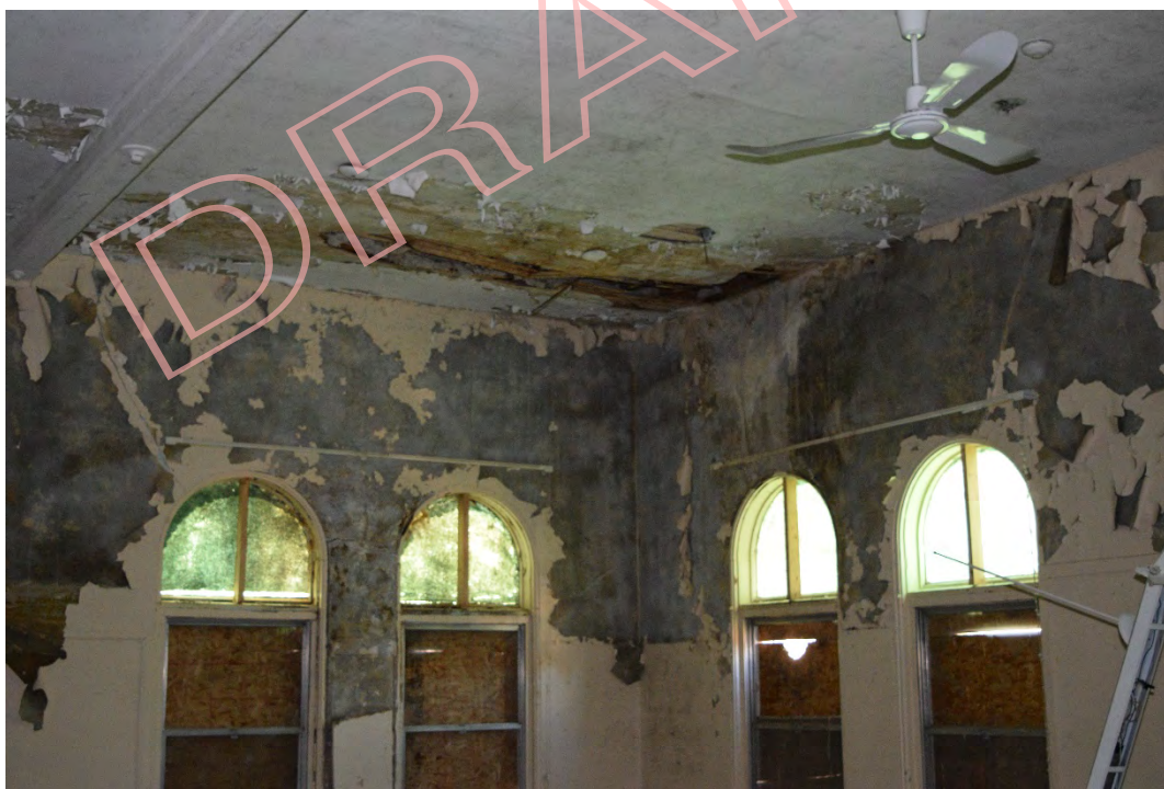
Figure 70: Water damage in the northwest corner of the west second-level classroom (May 2016).
