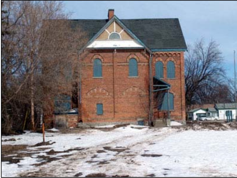
Figure 17: South façade, March 15, 2007.
