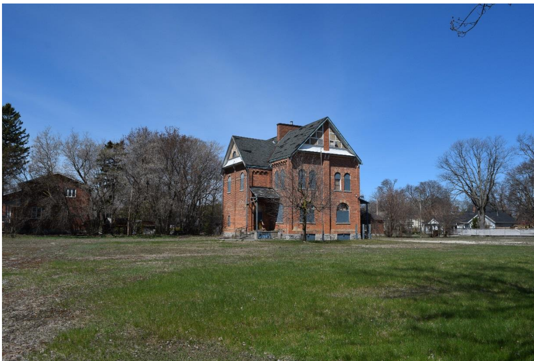
Figure 13: View of the property facing northwest (April 2016).
