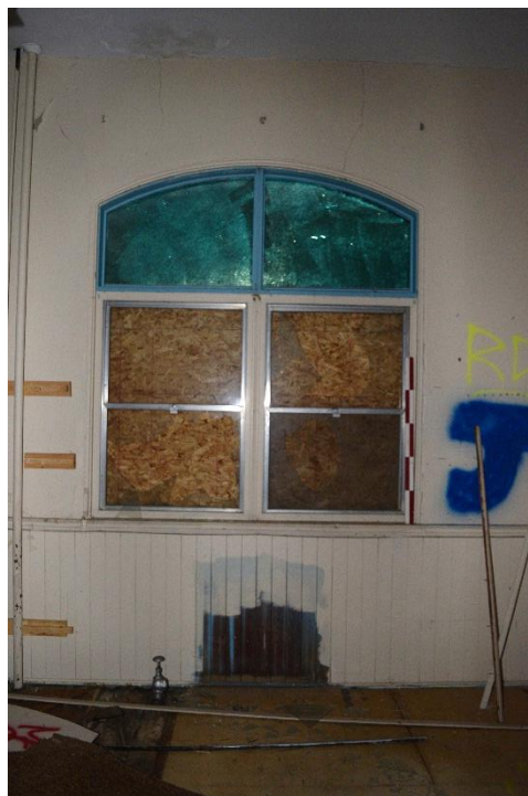
Figure 56: Former hot-water radiator location, wainscoting, chair rail, and window trim in the east first-level classroom (May 2016).
