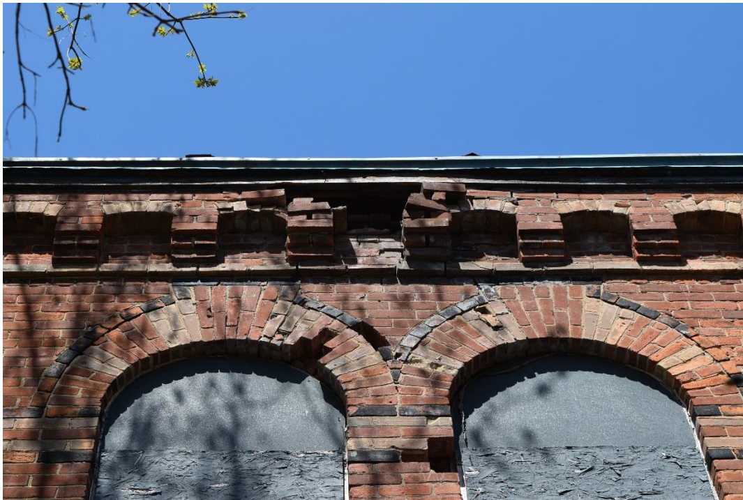
Figure 71: Missing and displaced section of arched corbel table, voussoir, and window column on the southwest façade of the main block (May 2016).
