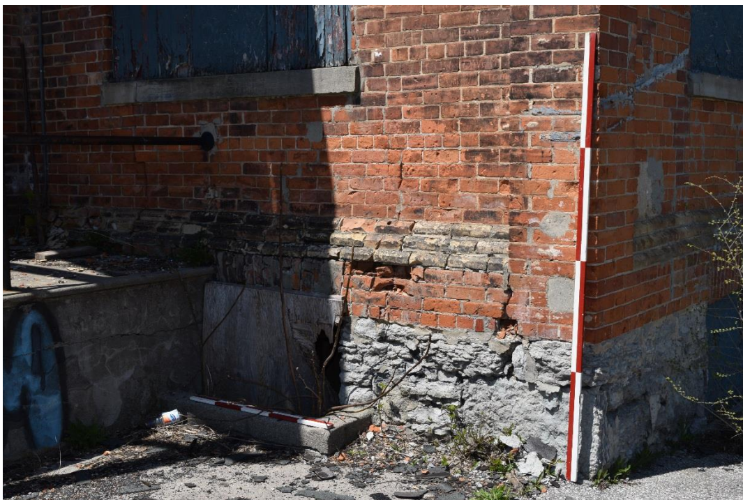
Figure 72: Erosion, exfoliation and spalling of the brick and stone construction on the southeast corner of the main block (May 2016).
