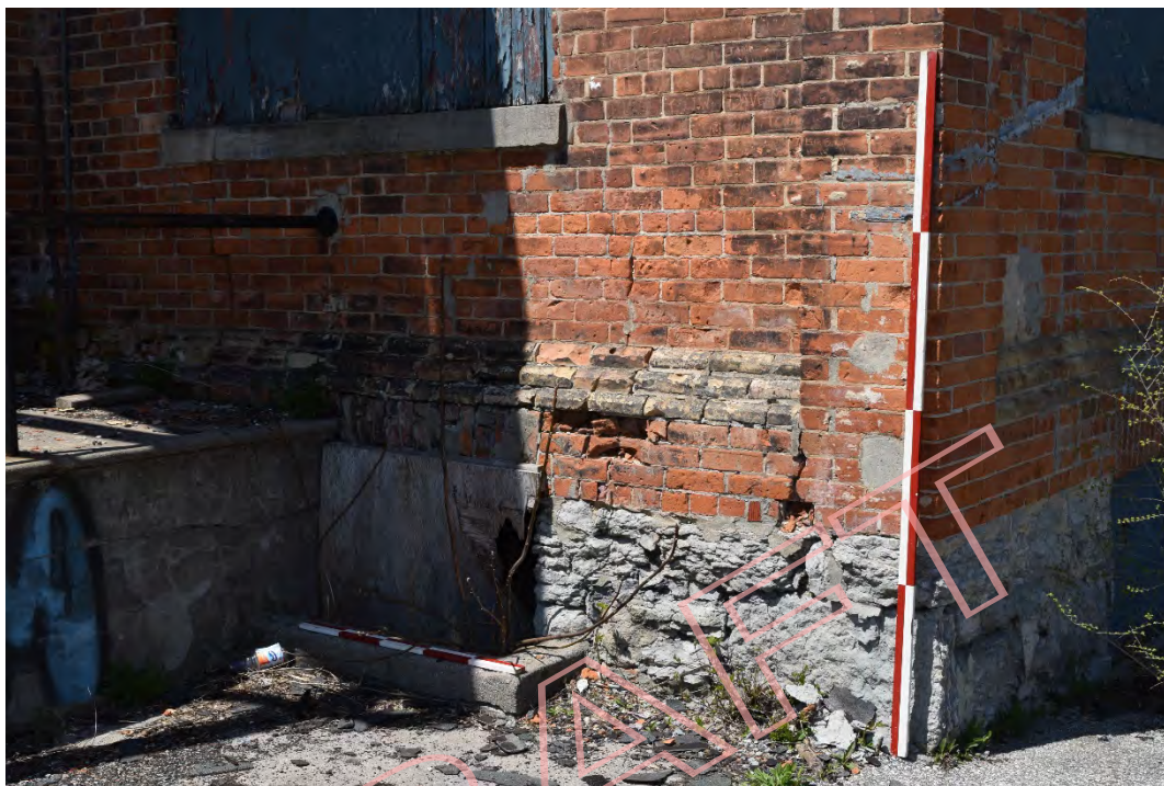
Figure 73: Erosion, exfoliation and spalling of the brick and stone construction on the southeast corner of the main block (May 2016).
