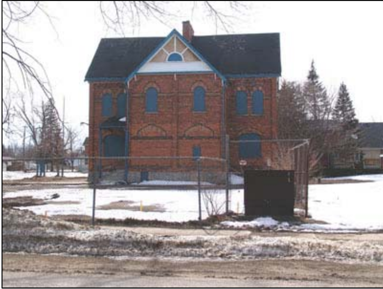
Figure 9: North façade of Annex, March 15, 2007.
