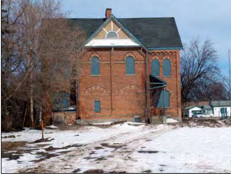
Figure 17: South façade, March 15, 2007.
