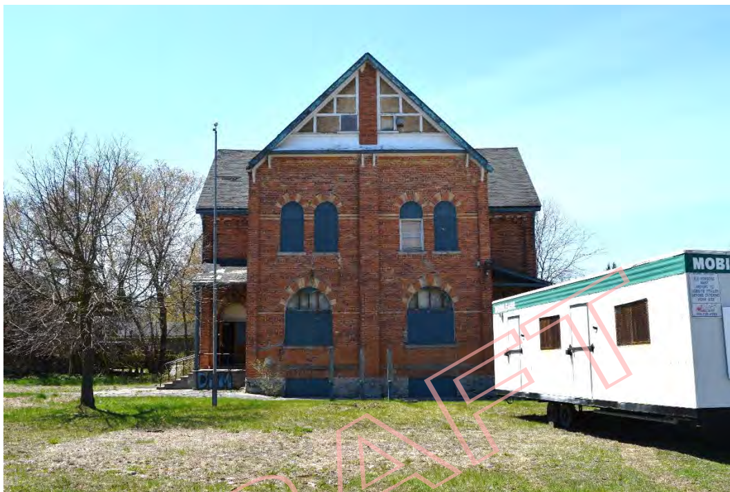
Figure 29: The east façade of the Annex (May 2016).
