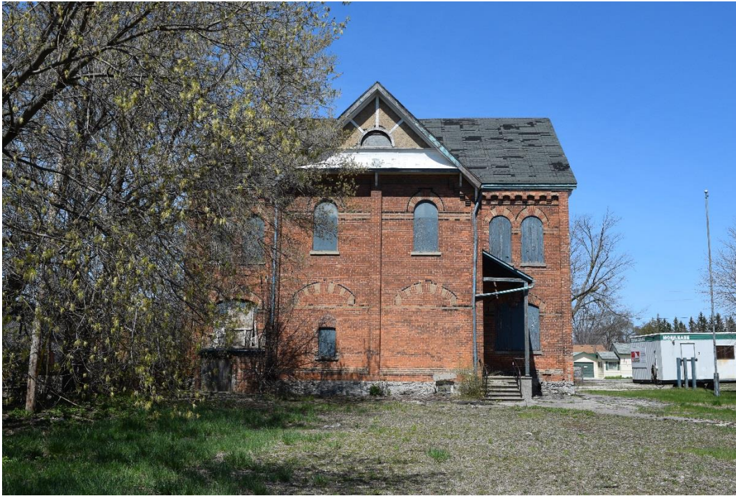
Figure 30: The south façade of the Annex (May 2016).
