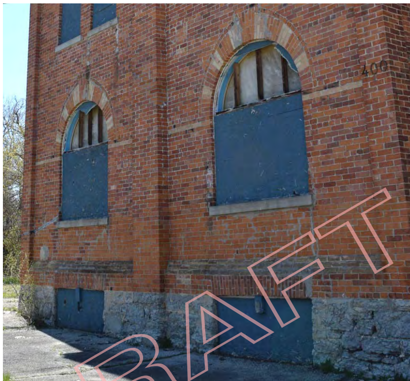
Figure 35: Diocletian windows on the east end wall of the main block (May 2016).
