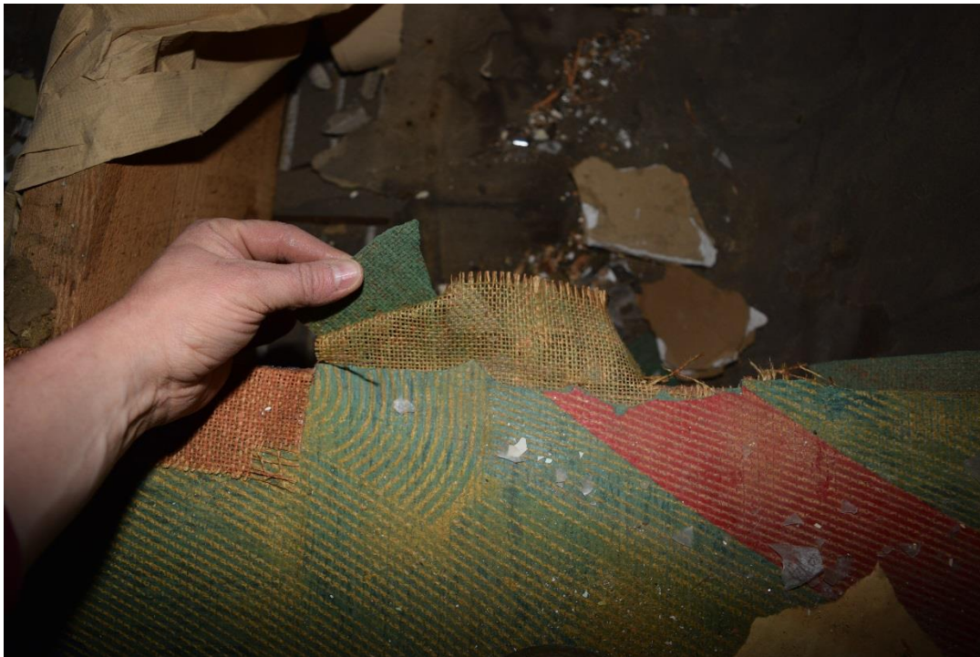
Figure 65: Painted sackcloth flooring in the second level classroom (May 2016).
