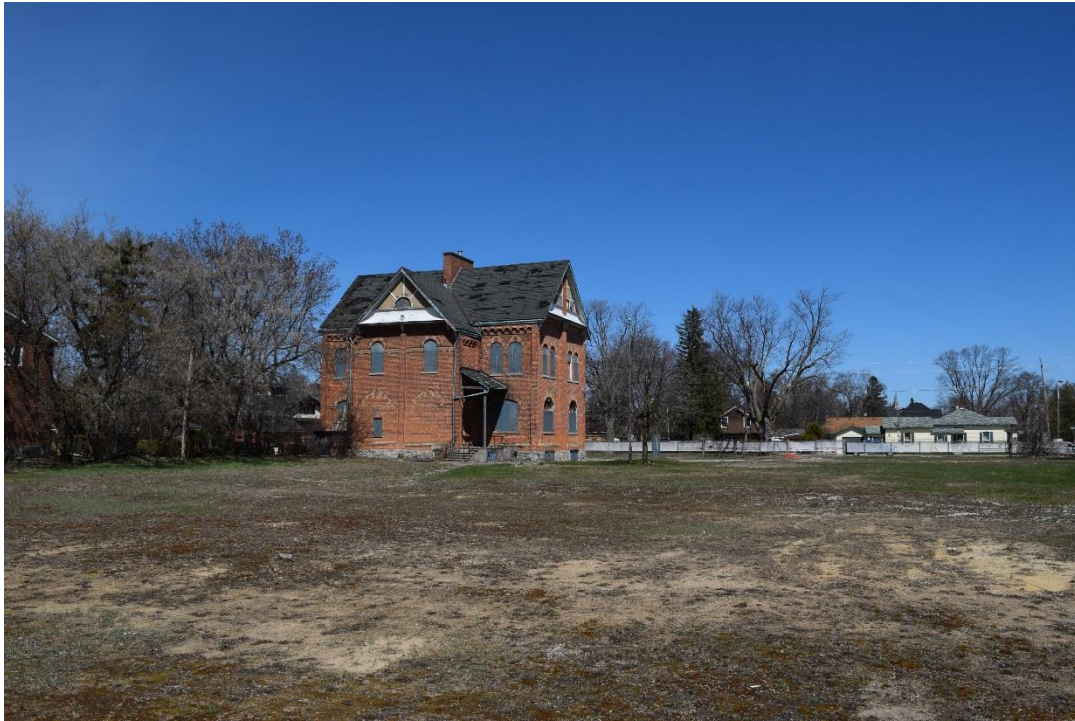
Figure 14: View from the property facing north (April 2016).
