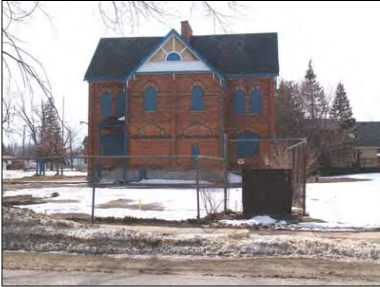
Figure 9: North façade of Annex, March 15, 2007.
