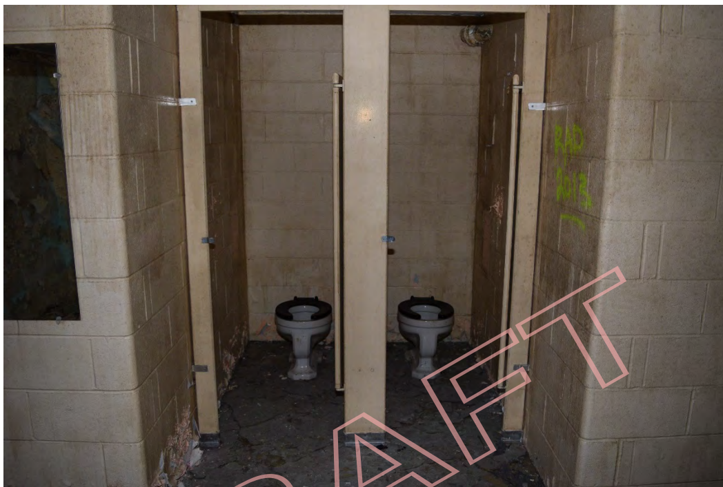
Figure 48: Toilet stalls in the 'Boys' bathroom (May 2016).
