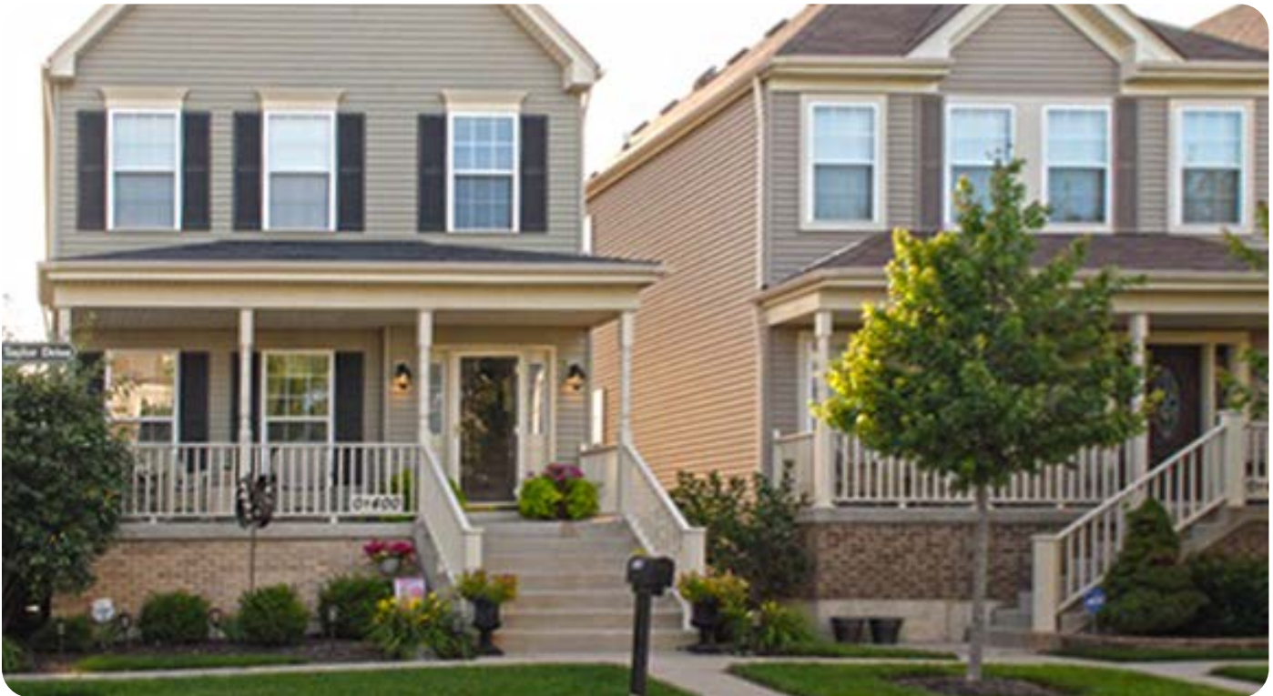
Elevated main front entrances used to address adverse grading conditions.
