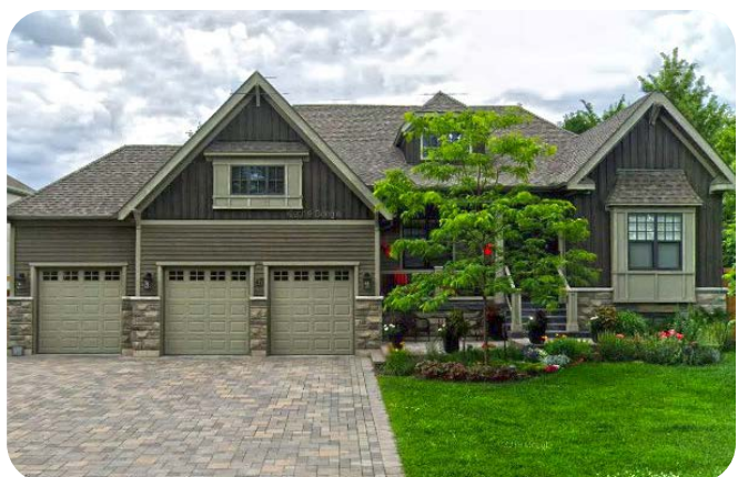
Existing built form on Saunders Street east of the site.
