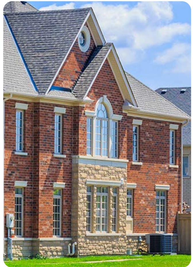
Example of architectural elements such as bays which add articulation to the building plane.
