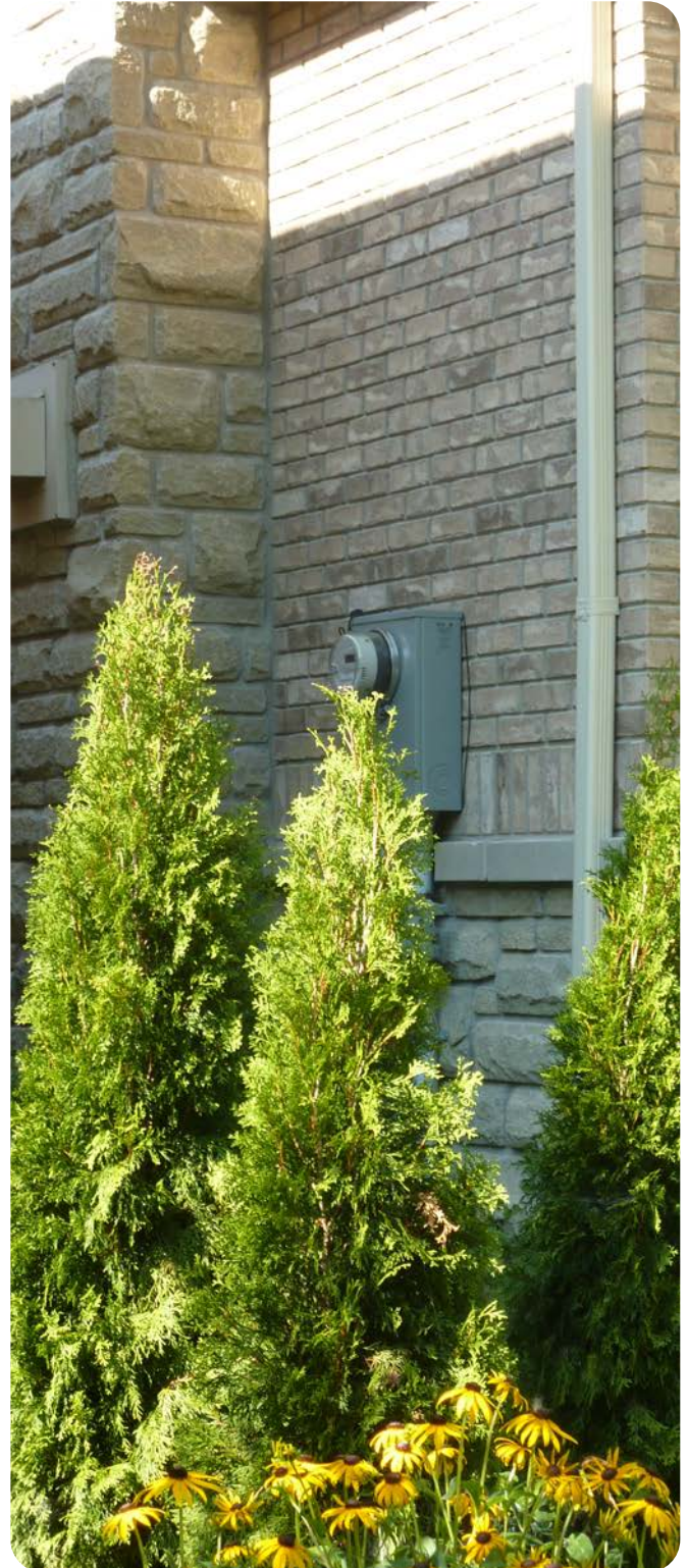
Example of appropriate placement and integration of utility metres.
