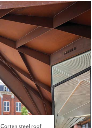
Corten steel roof
