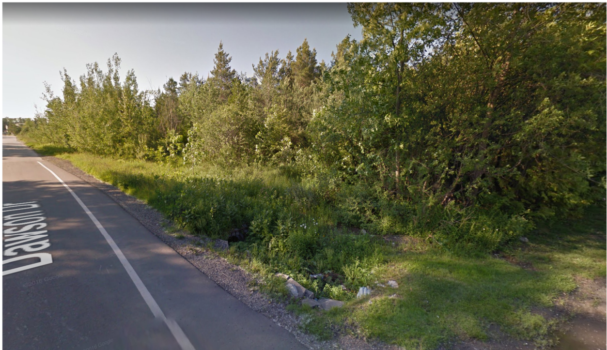
Dawson Drive – View Towards North
