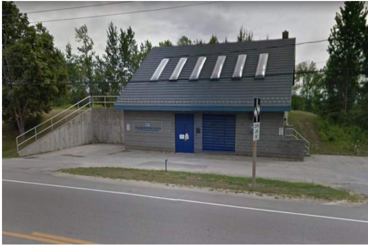
WATER RESERVOIR - NORTH OF SITE
