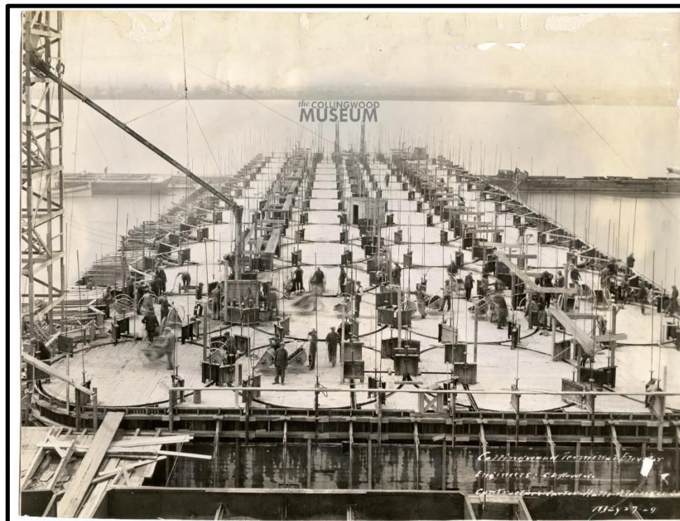
Plate 33: Collingwood Terminals During Concrete Pouring, May 27, 1929 (Facing Southwest; Provided by the Town of Collingwood)
