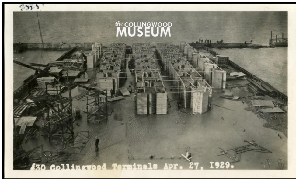
Plate 23: Collingwood Terminals Under Construction Showing Cribbing, April 27, 1929 (Facing Southwest; Provided by the Town of Collingwood)
