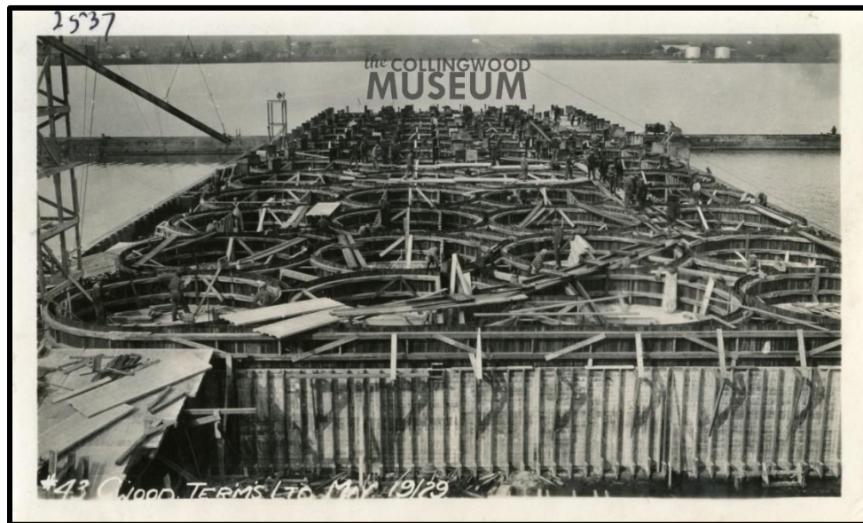
Plate 32: Collingwood Terminals During Concrete Pouring Showing Cylindrical Cribbing, May 19, 1929 (Facing Southwest; Provided by the Town of Collingwood)
