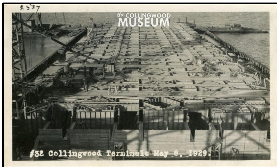
Plate 26: Collingwood Terminals Prepared for Concrete Pouring, May 8, 1929 (Facing Southwest; Provided by the Town of Collingwood)
