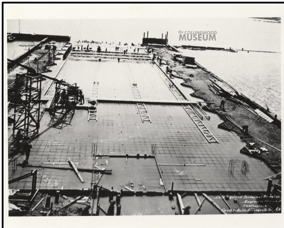
Plate 20: Pouring Basement Floor of Terminals, 1929 (Facing Southwest; Provided by the Town of Collingwood)
