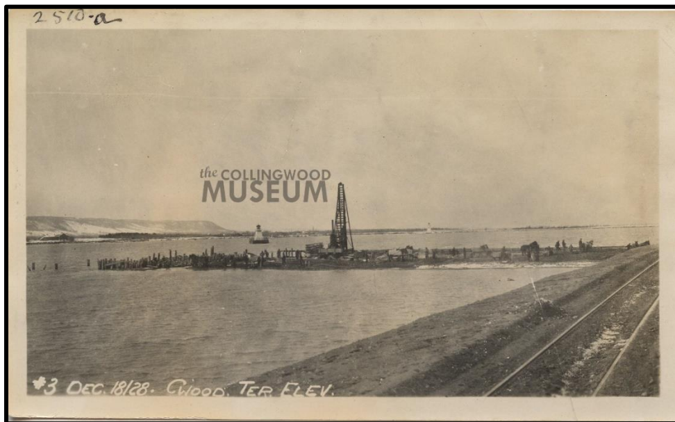
Plate 14: Driving Piles for Terminals Foundation, December 18, 1928 (Facing Northwest; Provided by the Town of Collingwood)
