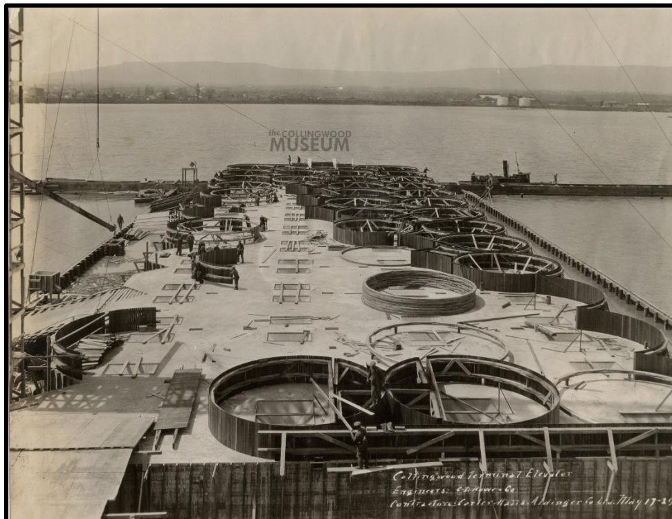
Plate 31: Collingwood Terminals During Concrete Pouring Showing Cylindrical Cribbing, May 17, 1929 (Facing Southwest; Provided by the Town of Collingwood)
