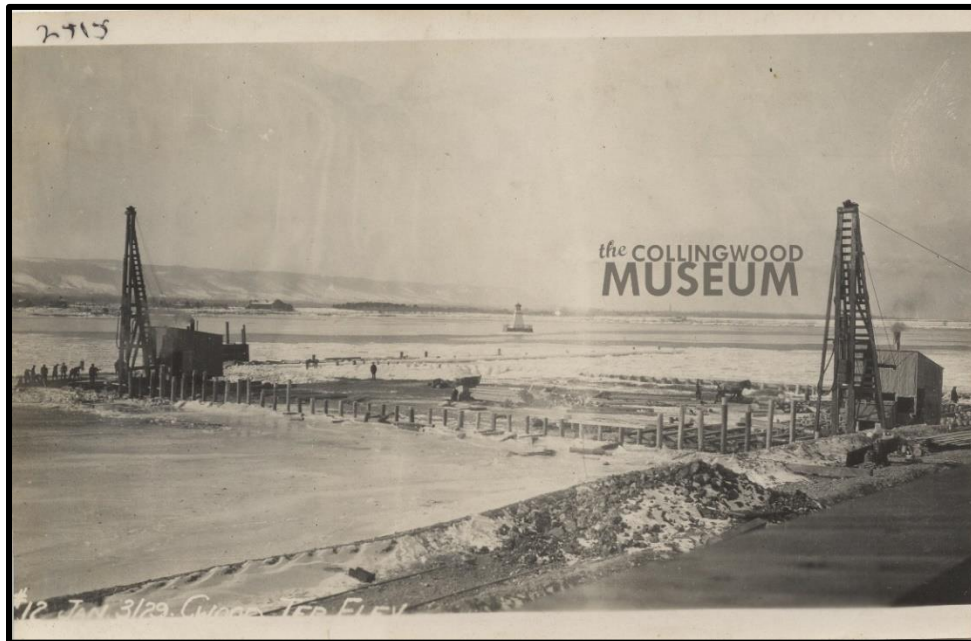
Plate 19: Pile Driving for Terminals Foundation, January 31, 1929 (Facing Northwest; Provided by the Town of Collingwood)
