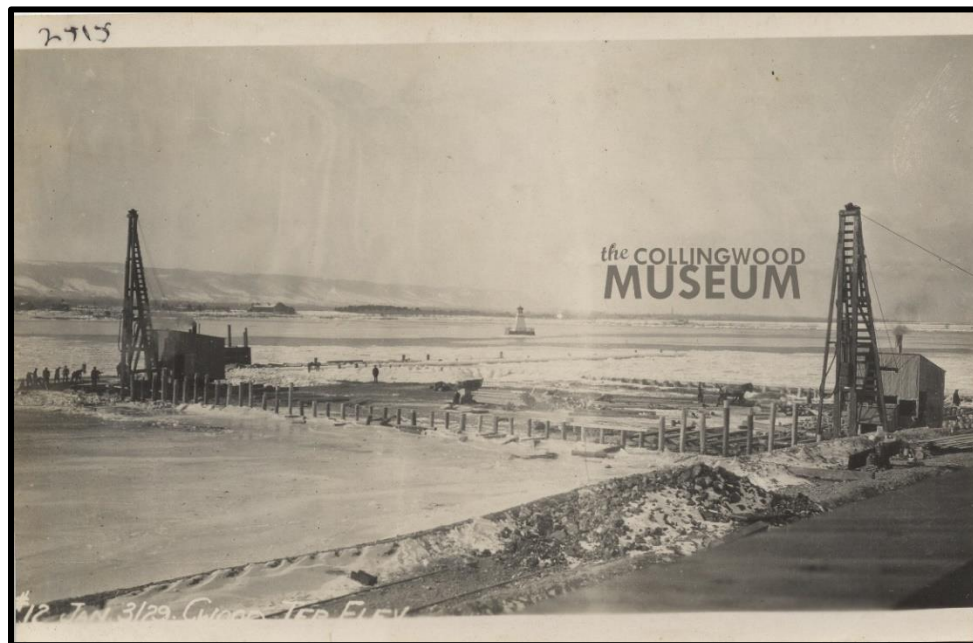
Plate 16: Driving Piles for Terminals Construction, January 3, 1929 (Facing Northwest; Provided by the Town of Collingwood)
