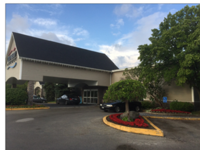
AMENITY BUILDING EXISTING MAIN ENTRANCE CANOPY
