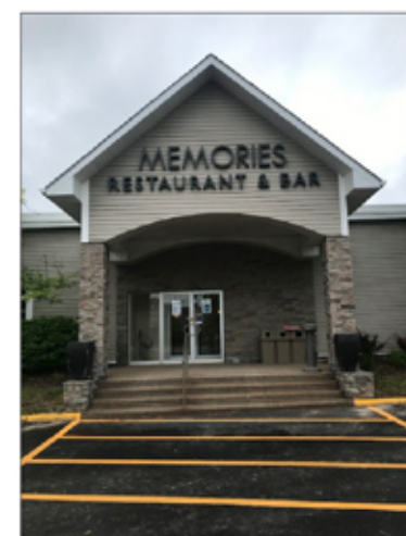
AMENITY BUILDING EXISTING SIDE ENTRANCE CANOPY
