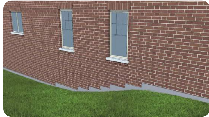
Foundation Wall at Sloping Grade
