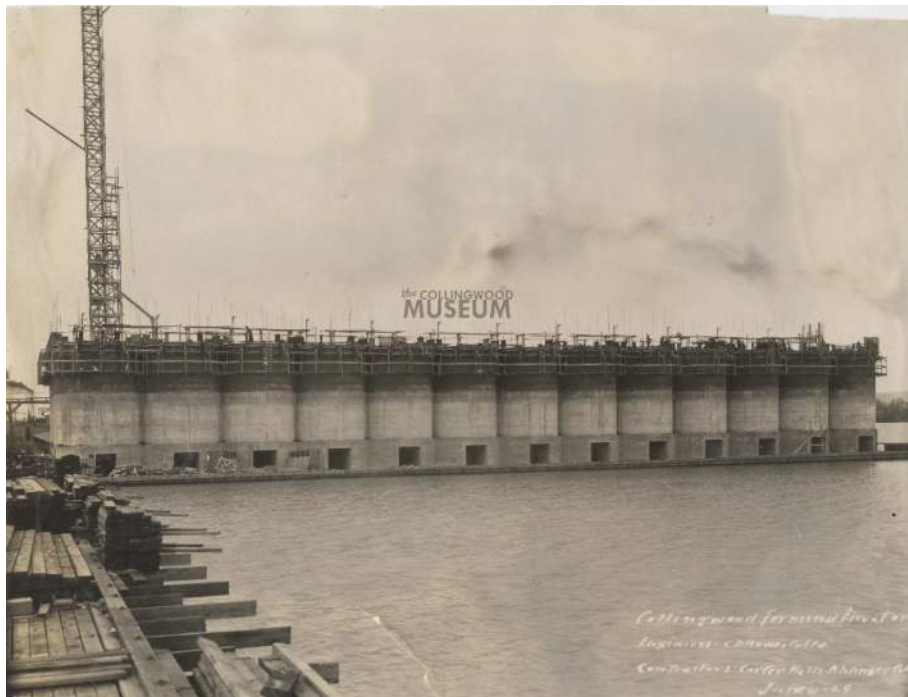
Figure 4: Silo Construction Level 2, June 1929
