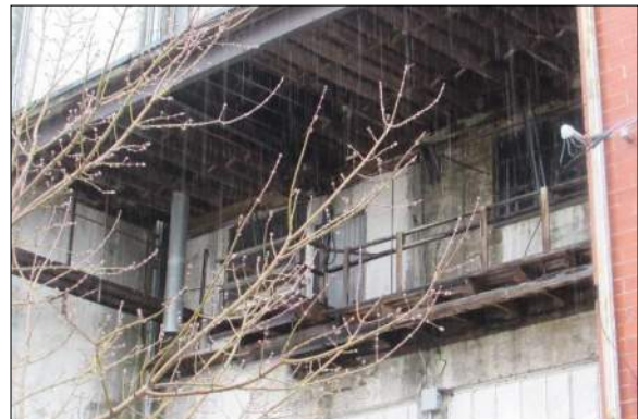
Figure 17a, b: Suspended Exterior Platform (Outside Second Floor of Bagging Room)
