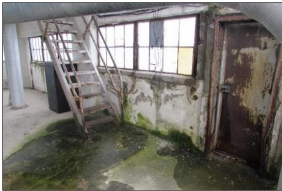
Figure 21a, b: Steel Stair to Shipping Tower Mezzanine in Poor Condition (Floor 4)
