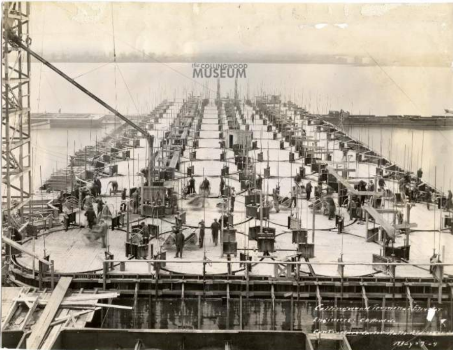
Figure 3: Silo Base, May 1929
