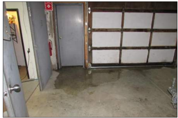
Figure 29a, b: Water Infiltration Under Overhead Doors in Rail Shed (Storage)
