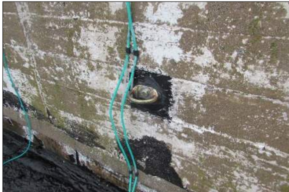
Figure 32a, b: Fall Arrest Anchor at Shipping Tower roof
