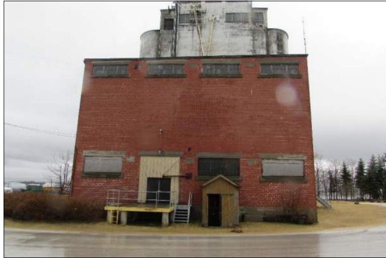
Figure 18: Exterior Shipping Platform
