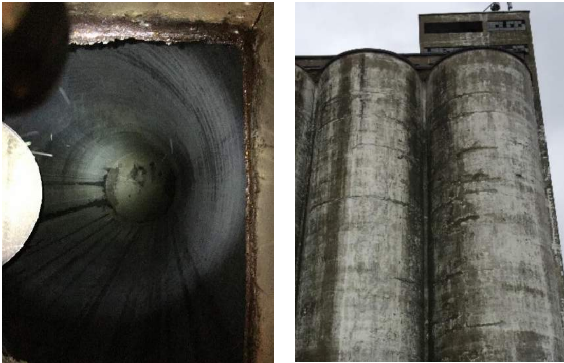
Figure 8 a, b: Interior and exterior of typical concrete silo
