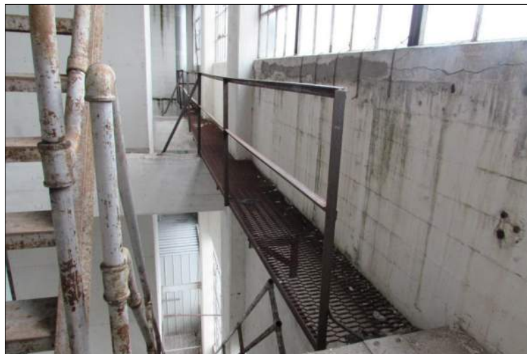
Figure 23: Service Platform from Floor 3 Mid-Landing of Shipping Tower
