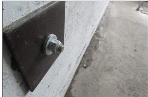
Figure 32a, b: Fall Arrest Anchor at Shipping Tower roof
