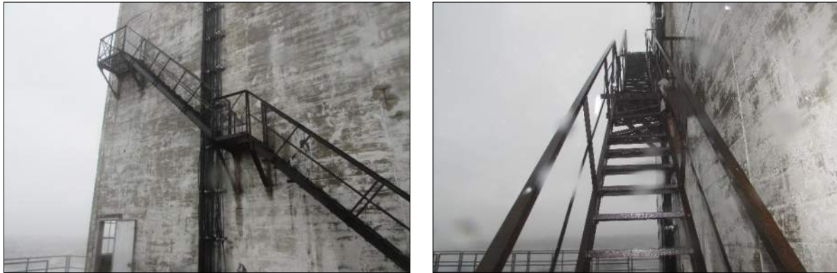
Figure 26a, b: Exterior Steel Stair Outside Marine Tower
