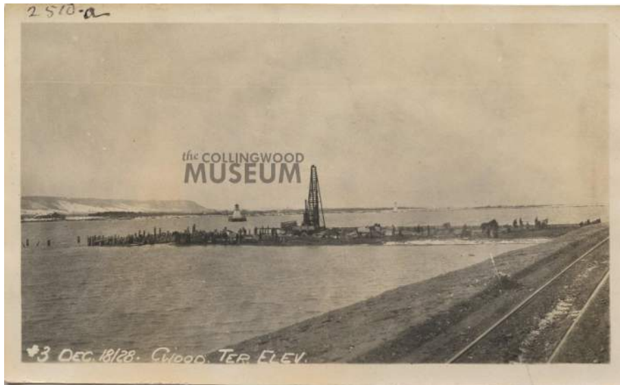
Figure 1: Pile Construction, December 1928
