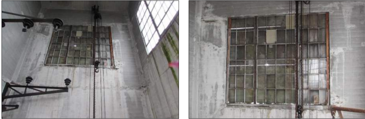
Figure 19a, b: Window at East End of Electrical Substation
