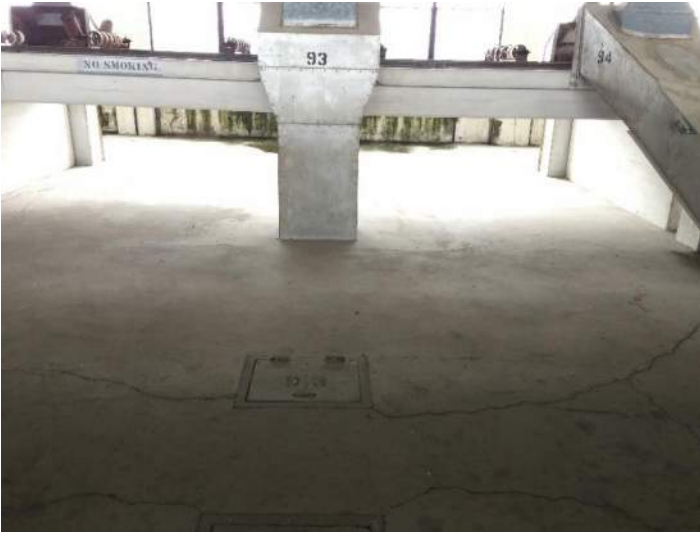
Figure 9 a, b: Silo Top Slab Cracking
