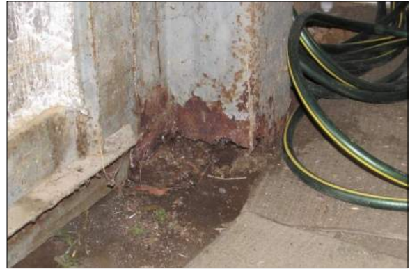
Figure 28a, b: Corrosion of Steel Door Jambs in Warehouse (Shop)
