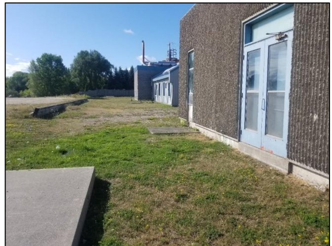
Photo 4: Visually confirmed disturbance (building footprint, underground utilities), facing south
