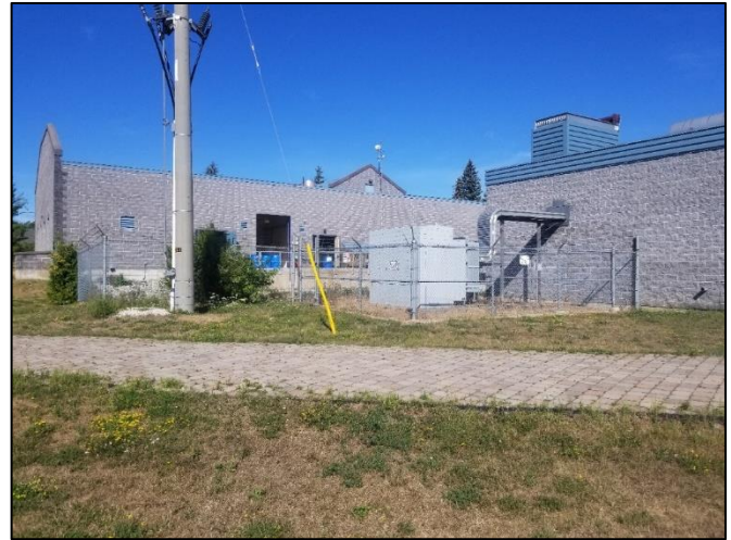
Photo 2: Visually confirmed disturbance (building footprint, underground utilities), facing north east
