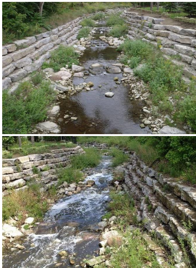
Figure 1. Example of previously installed vortex rock weir and pool system with armoured stone retaining walls
