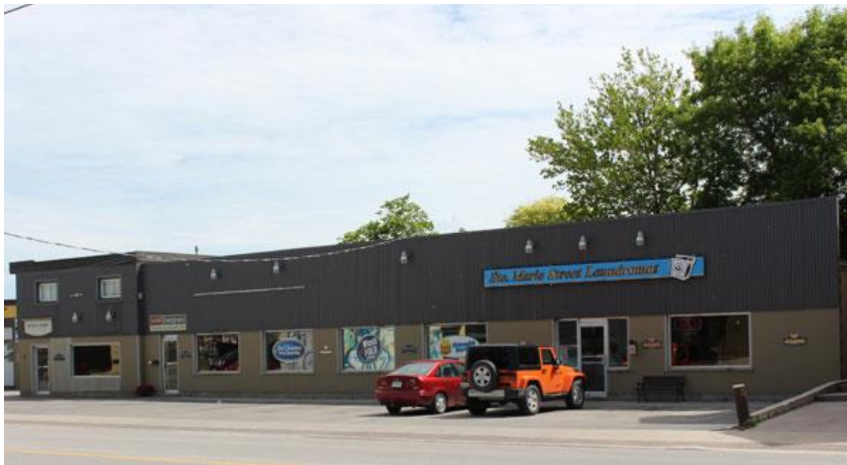
Figure 22: 7 Ste Marie Street (photo from Heritage Collingwood)
