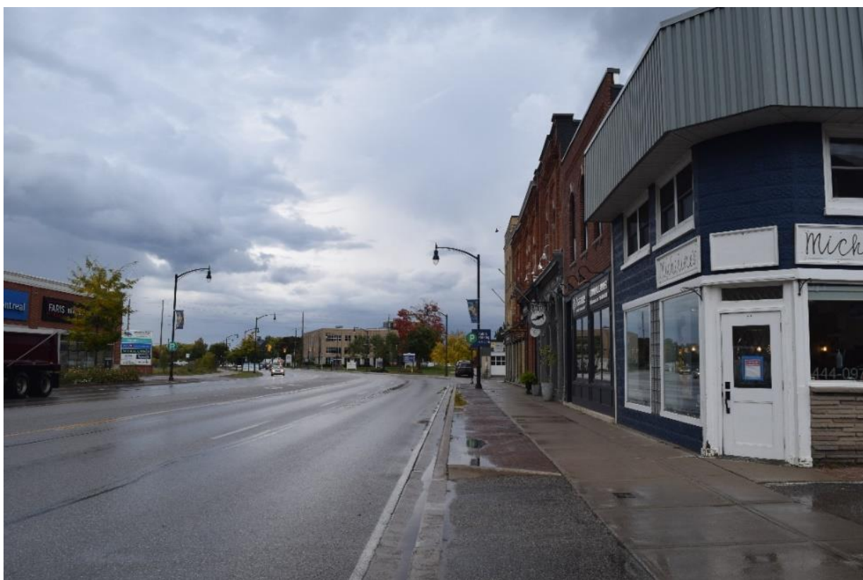
Figure 18: 12 Huron Street, facing east
