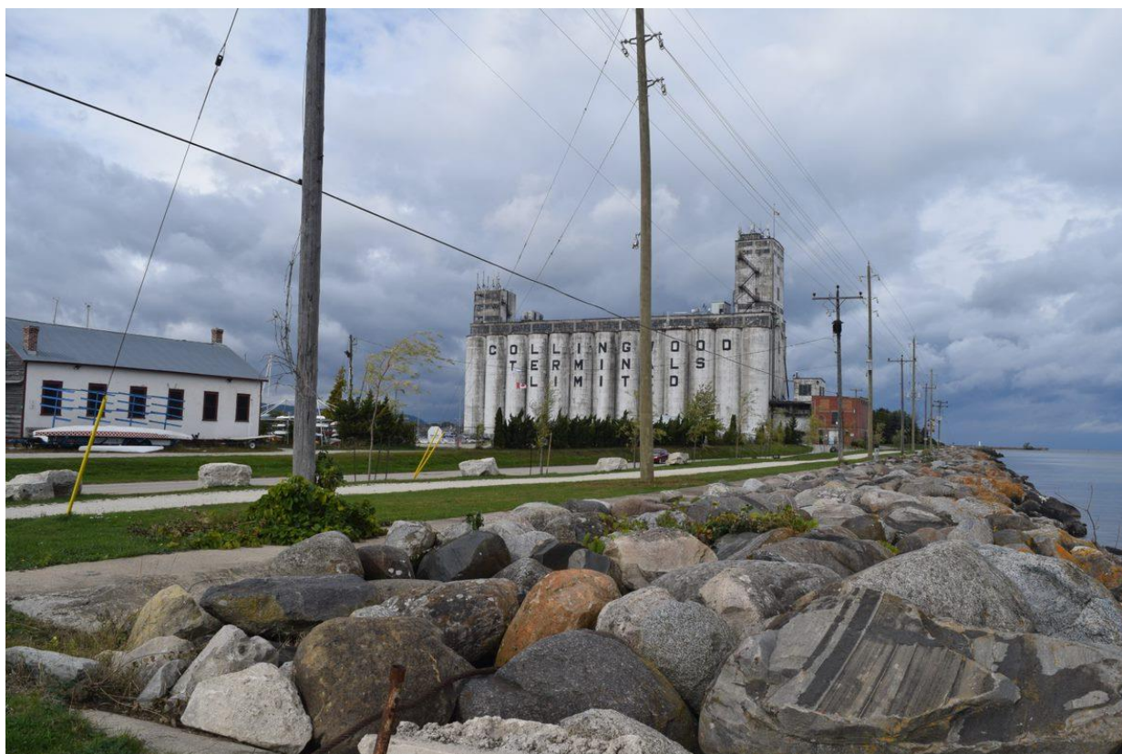
Figure 25: View north of the Collingwood Terminals Grain Elevator.
