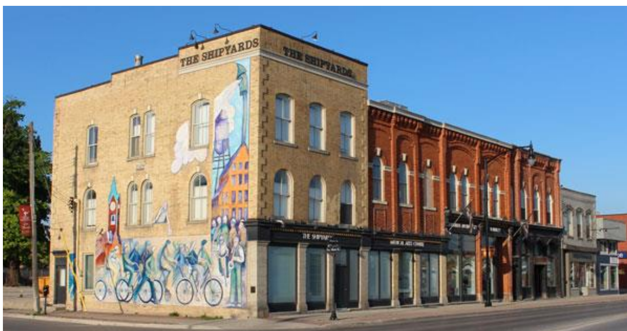
Figure 21: 28 Huron Street (photo from Heritage Collingwood)
