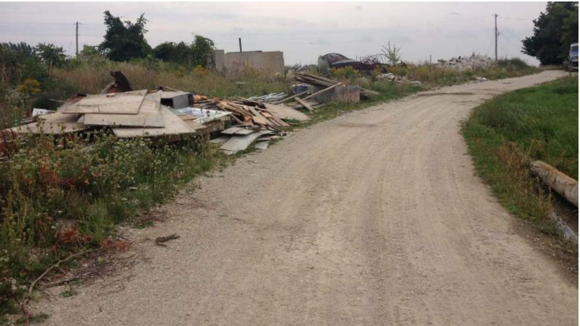
Photograph 6: View facing east of the north barn foundation and debris piles taken on September 10 th 2014.
