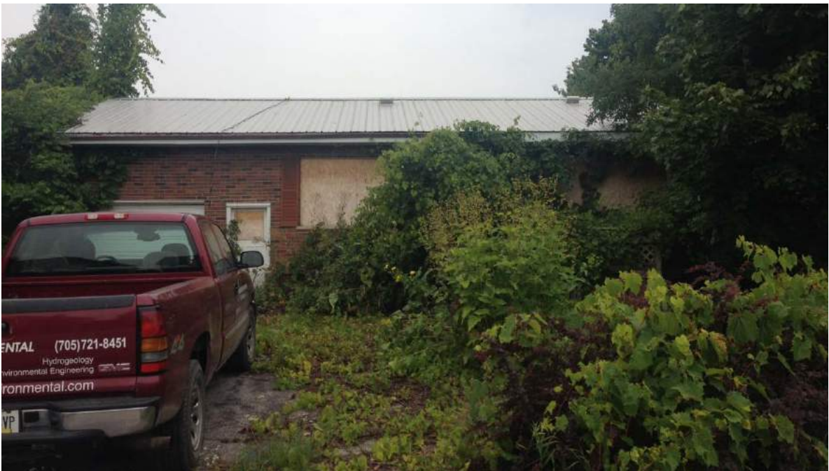
Photograph 10: View facing west of the abandoned residence taken on September 10 th 2014.
