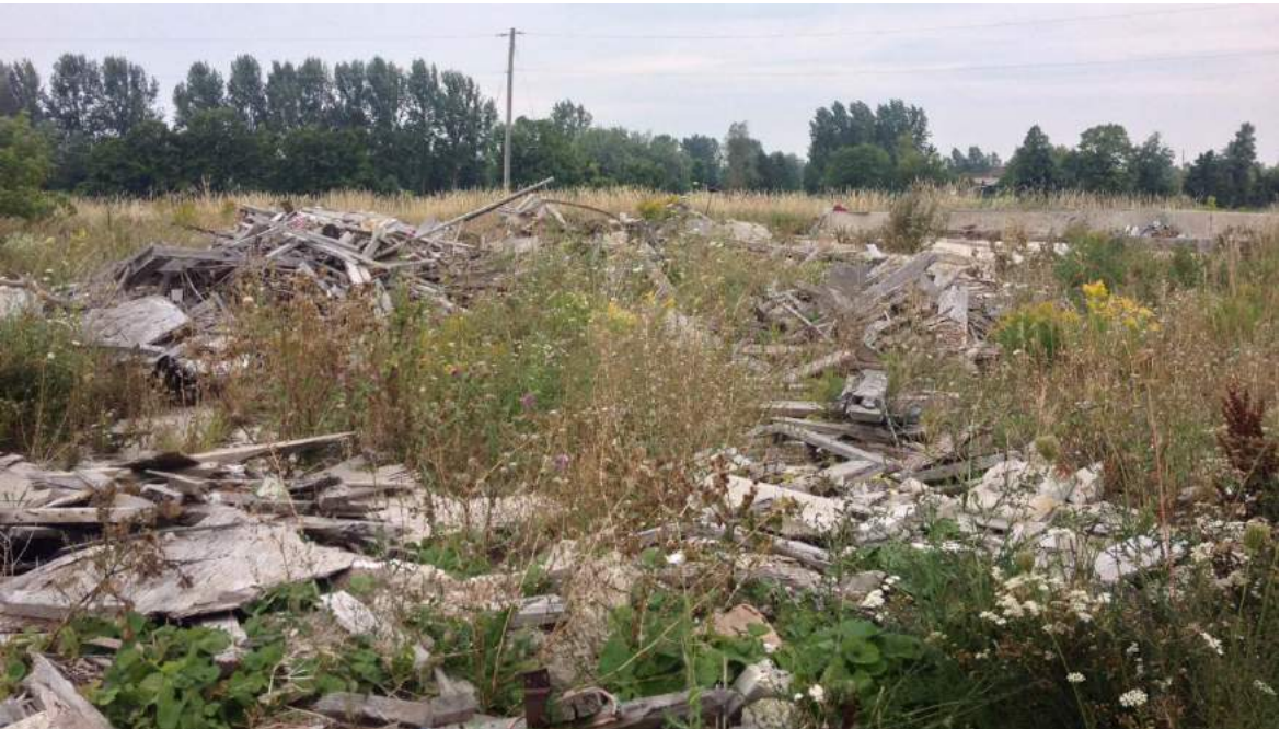
Photograph 8: View facing north of the wood and concrete piles taken on September 10 th 2014.
