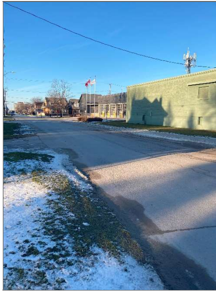
Photograph 13 – Cold storage warehouse and paramedic station west of Site, viewed from the southwest.
