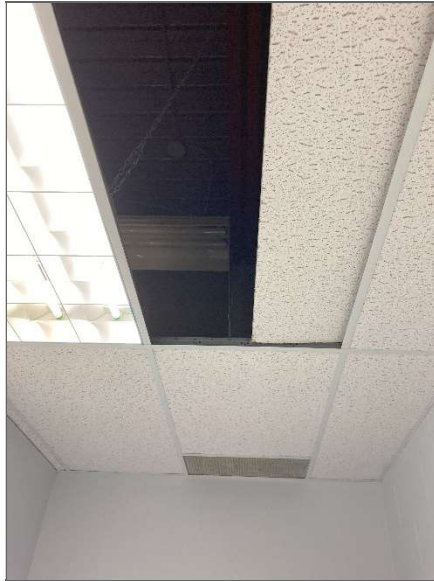
Photograph 7 – Original fluorescent lighting above current suspended ceiling.
