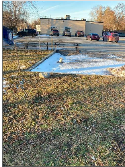
Photograph 3 – Looking north at south wall of on-Site building and heaved casing of on-Site flushmount well.
