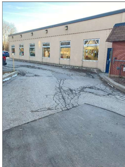
Photograph 2 – West wall of on-Site building viewed from the northwest.
