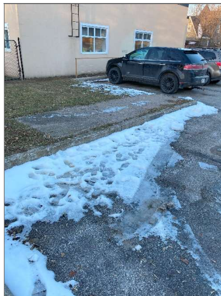
Photograph 4 – Concrete pad near southwest corner of on-Site building.
