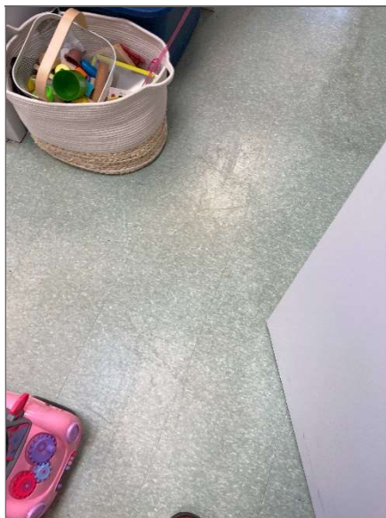
Photograph 8 – Vinyl tiles, limited use in southern portion of building.
