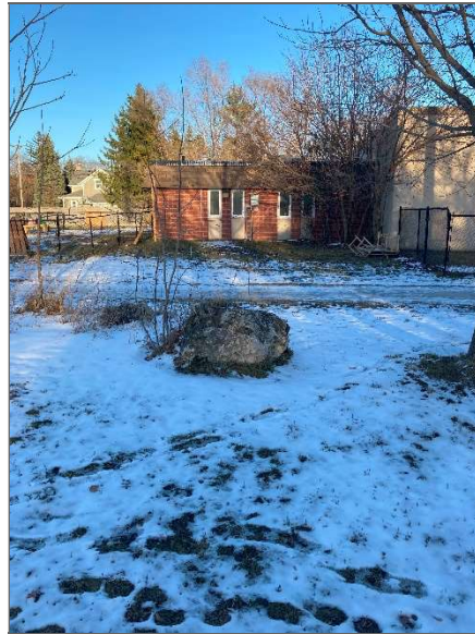
Photograph 5 – Looking west at northern portion of on-Site building.
