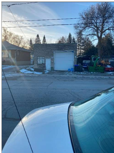
Photograph 14 – Old garage west of cold storage warehouse, looking west.
