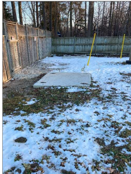
Photograph 10 – Concrete pads west of the transformer compound, looking south.
