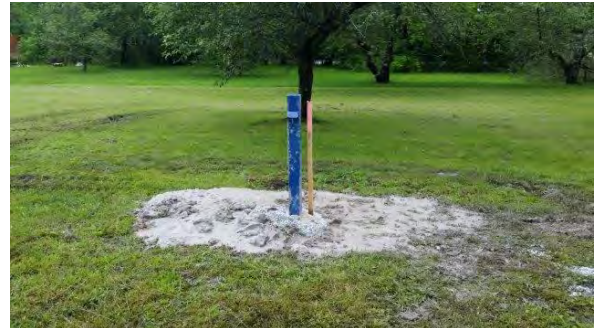
14. View of monitoring well installed during Geotechnical Investigation.
