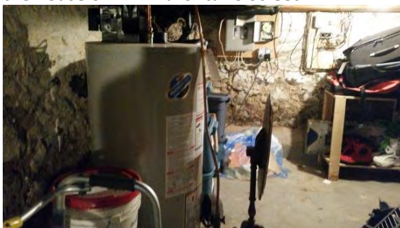
23. View of basement of the house on 774 Hurontario Street.
