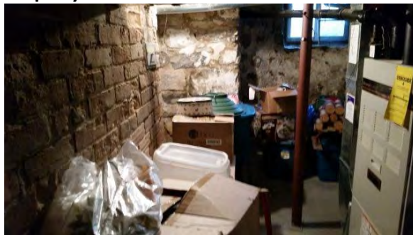
20. View of basement of the house on 774 Hurontario Street.
