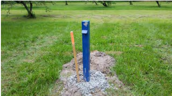
15. View of monitoring well installed during Geotechnical Investigation.
