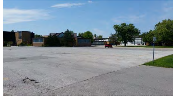
26. View of high school to the north and the location of an underground heating fuel oil tank.
