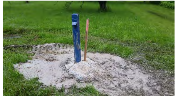
16. View of monitoring well installed during Geotechnical Investigation.
