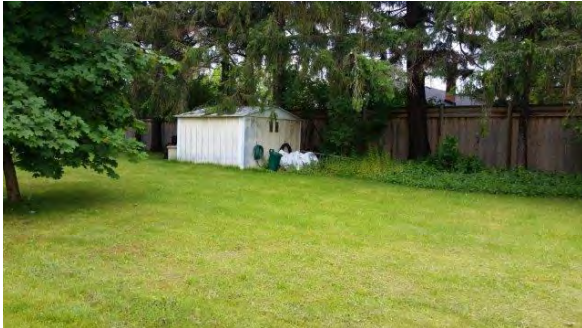
11. View of outdoor storage shed in backyard of 774 Hurontario Street, facing south.
