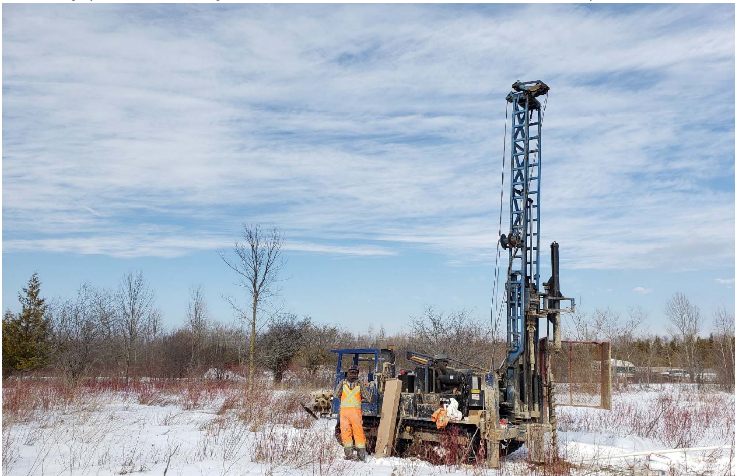
Photograph 4: View of the installation of borehole BH3 located in the orchard area at the north side of the Site.
