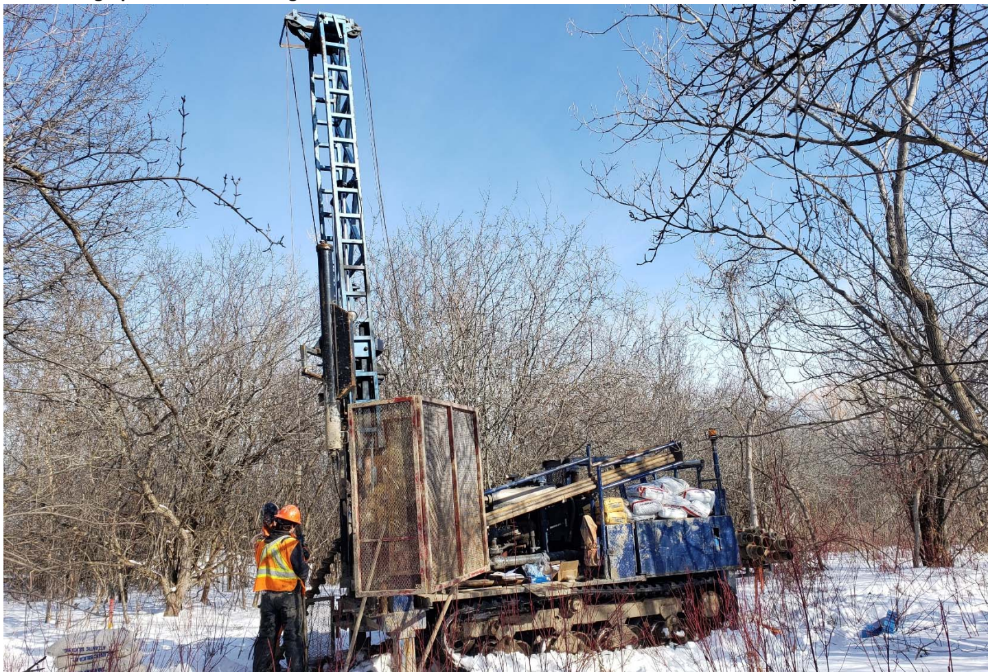
Photograph 2: View of the installation of borehole BH1 located in the orchard area at the east side of the Site.
