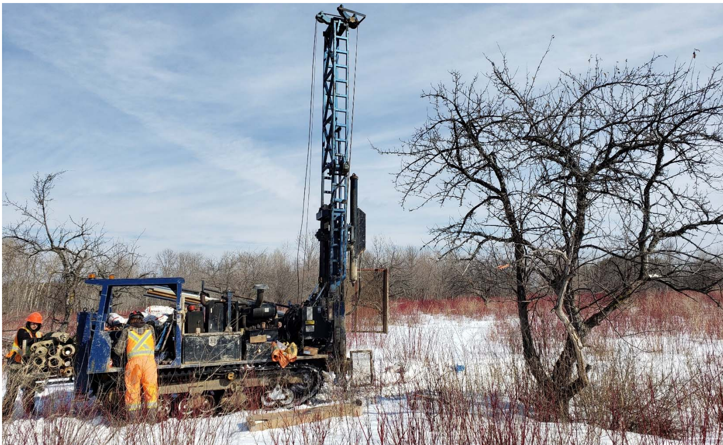
Photograph 5: View of the installation of borehole BH2 located in the orchard area at the east side of the Site.
