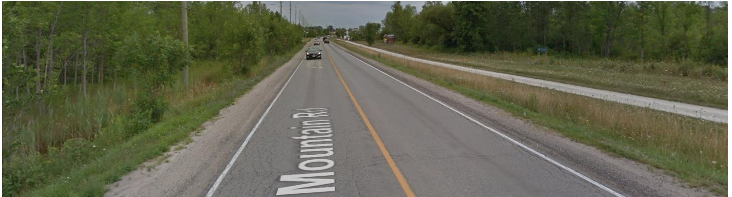
Looking east along Mountain Road from the frontage of the site
