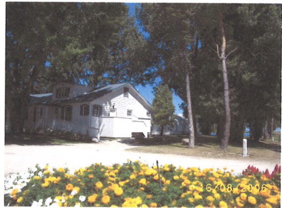
Plate 10 South Façade of Garage with Gravel Path facing Northeast
