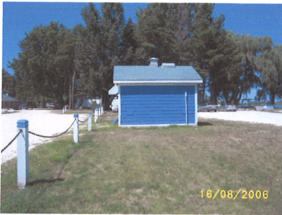
Plate 7 Pump House near East Edge of Boundary facing North
