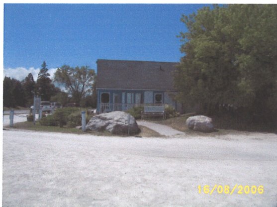
Plate 5 E Façade of Cranberry Marina Office with Parking Area facing West
