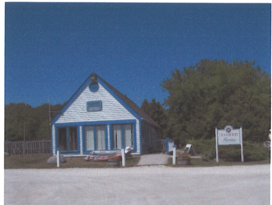
Plate 4 South Façade of Cranberry Marina Office facing North
