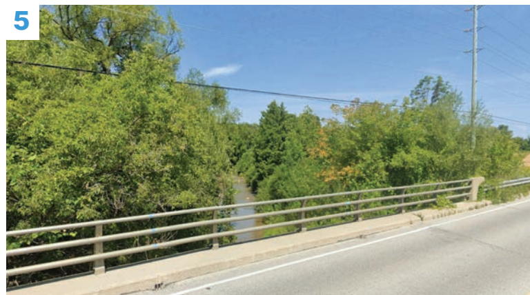
View of the Pretty River from Poplar Sideroad
