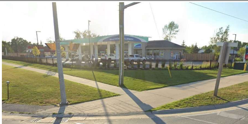
Photo #3: Gas station at 7618 Poplar Sideroad (~30 m west of Site).
