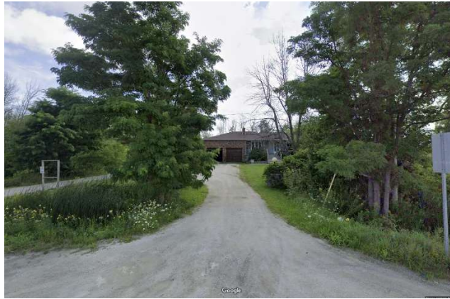
Photo #4: Looking east at 853 Hurontario Street residential house (Google Earth image)
