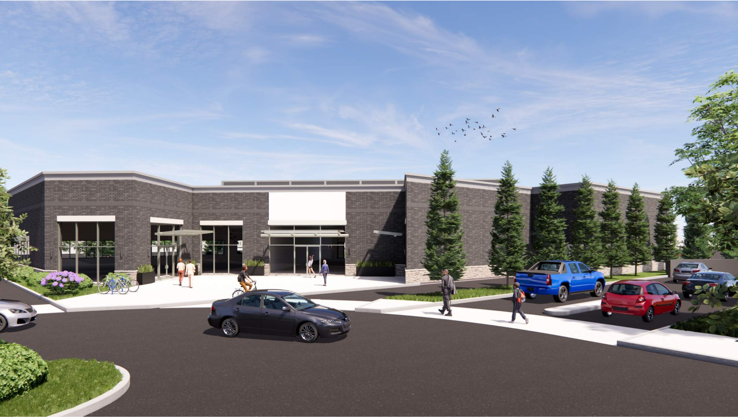
VIEW TOWARDS COMMERCIAL BUILDING
