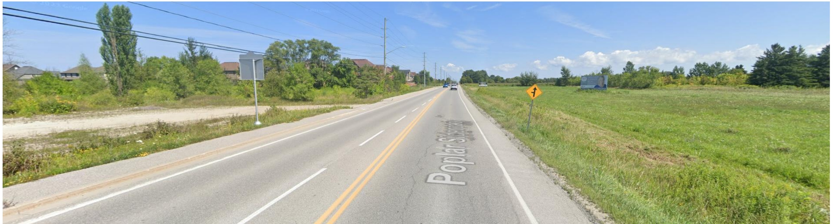
Looking east on Poplar Sideroad from proposed Access 2
