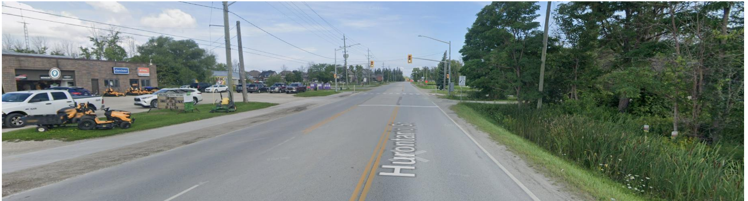
Looking north on Hurontario Street from proposed Access 1
