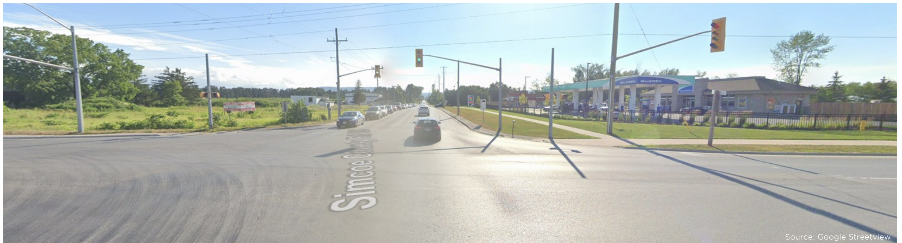
Looking west on Poplar Sideroad/County Road 32 from intersection with Hurontario Street/County Road 124
