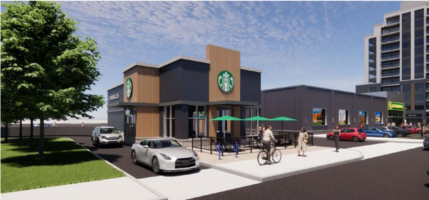
Pedestrian-friendly streetscape with articulated façades and unified design character.
