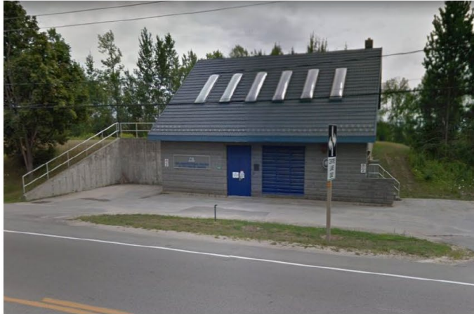
WATER RESERVOIR - NORTH OF SITE
