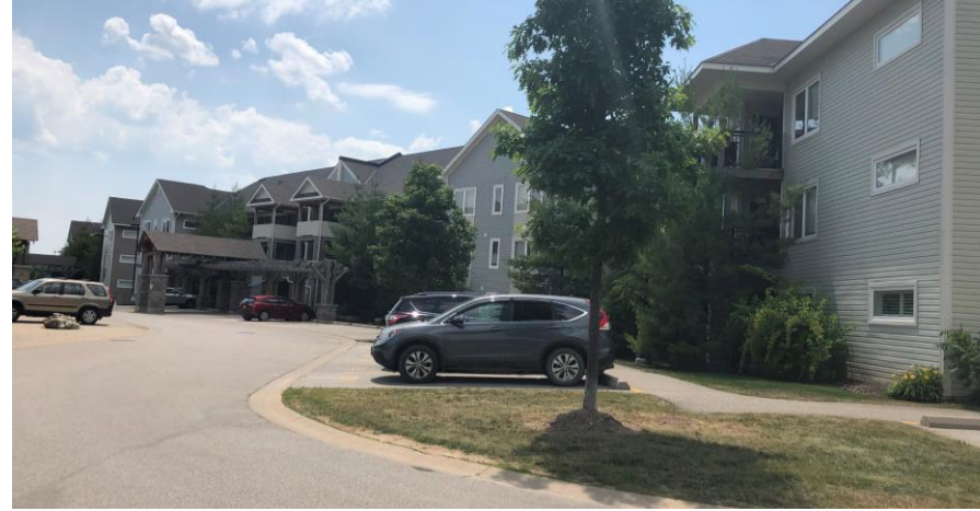
TOWNHOMES – SOUTH (Wyldewood)
