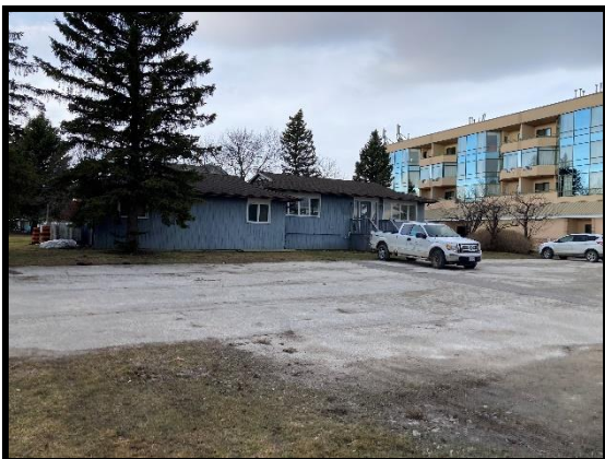
Image 9: Disturbed Area (March 5, 2024; Facing West)
