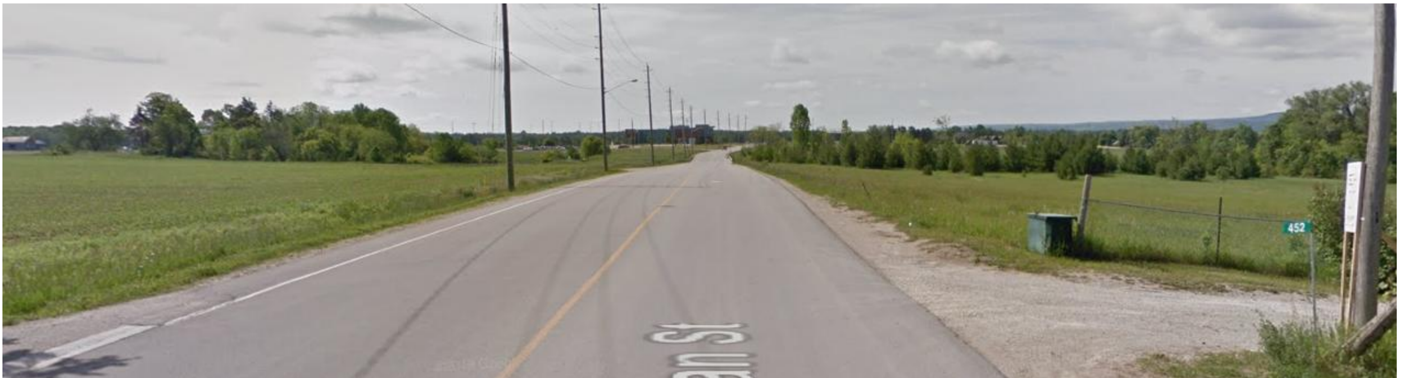
Looking south on Raglan Street from proposed site access
