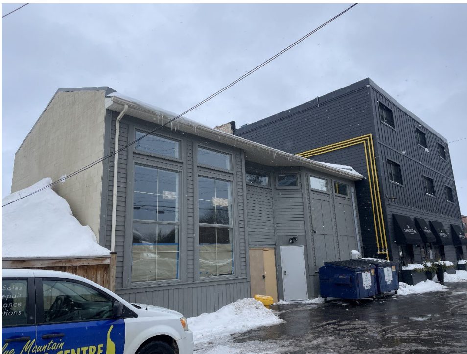
Figure 17: Rear (west) elevation of 168 Hurontario St. at left with 172 Hurontario St. at right.
