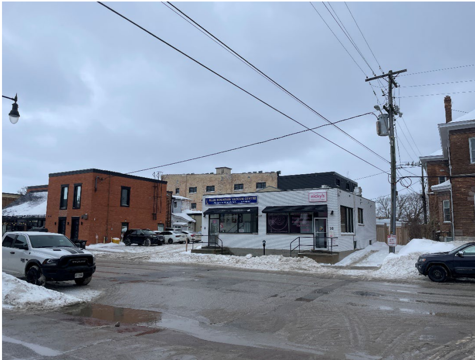
Figure 32: North elevation of 172 Hurontario St. as visible looking south from Third St.
