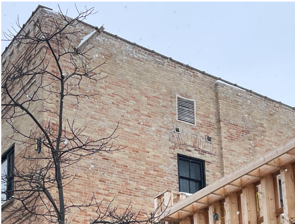
Figure 14: Detail of north elevation showing original brick arch above the window.
