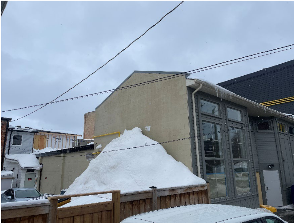
Figure 18: Northwest elevation of 168 Hurontario St, showing construction on the roof.
