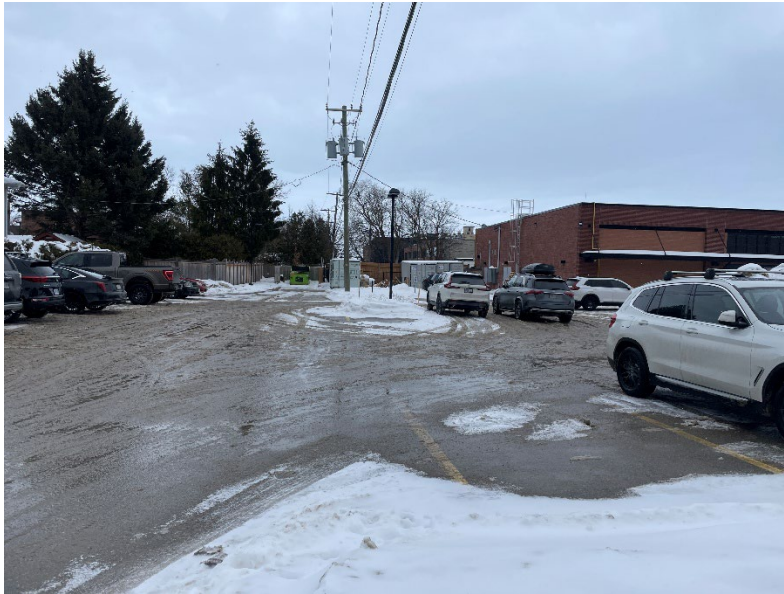
Figure 34: South elevation of 172 Hurontario St. as visible looking north from Fourth St.
