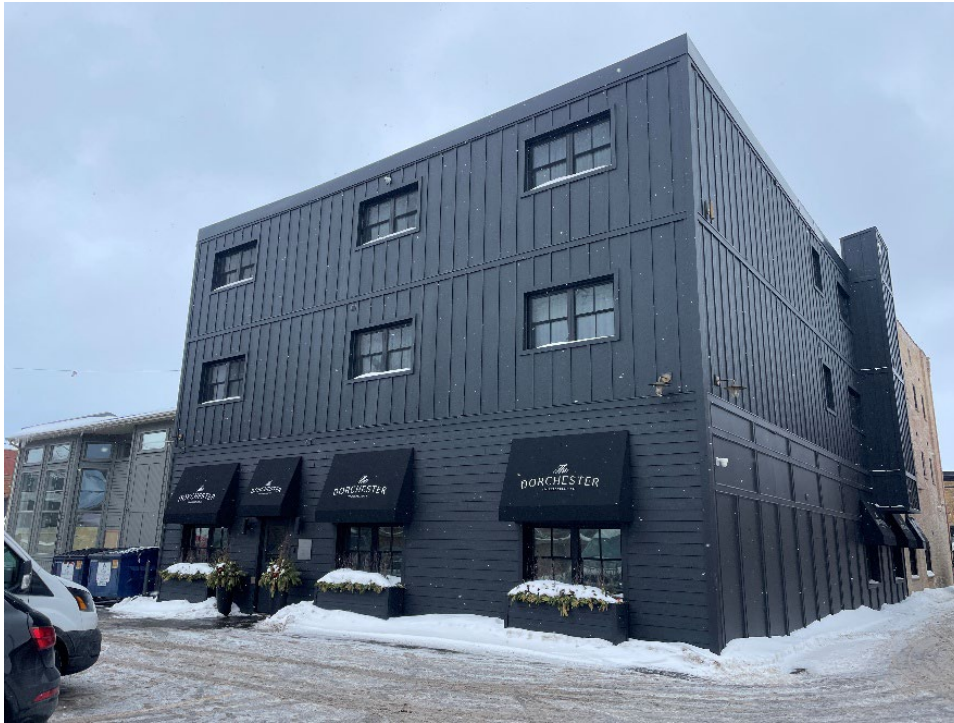
Figure 15: Rear (west) elevation, with 172 Hurontario St. at right and 168 Hurontario St. at left.
