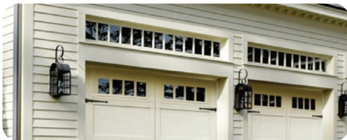
Example of Added Windows above the Garage Doors to Mitigate Excess Masonry above the Garage Doors
