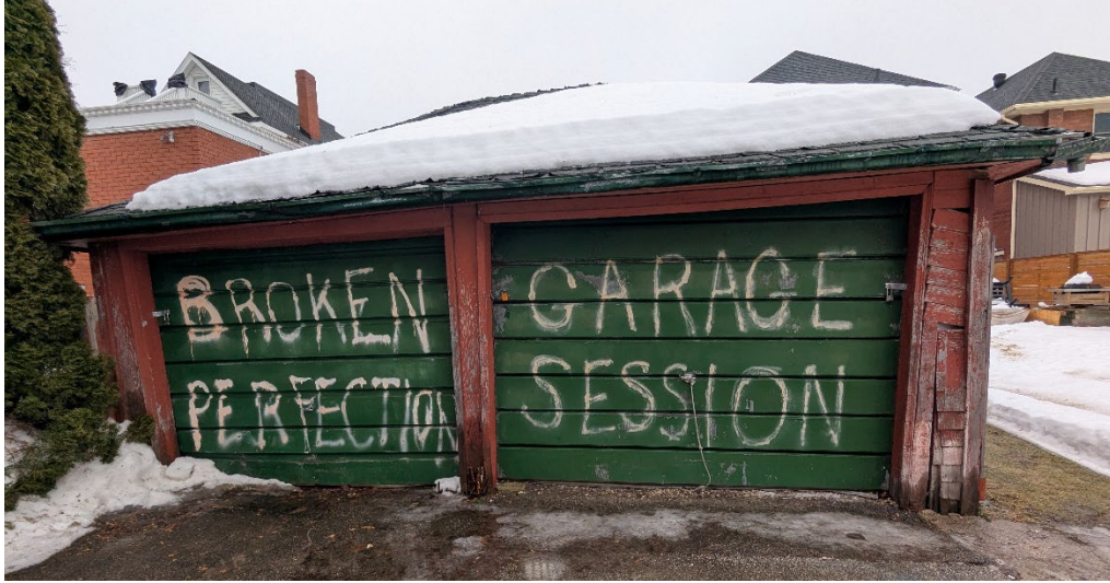
Rotted and water damaged wood noted along the base of the structure and roofline at the north and east elevations above, along with badly deteriorated shingles at the roof peak.
