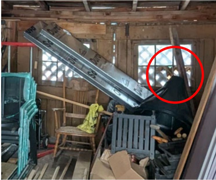
Broken window panes noted with a red circle above.
