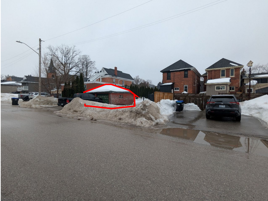
Photo 10: View west across Tremont Lane towards the subject property. The location of the existing garage is noted in red.
