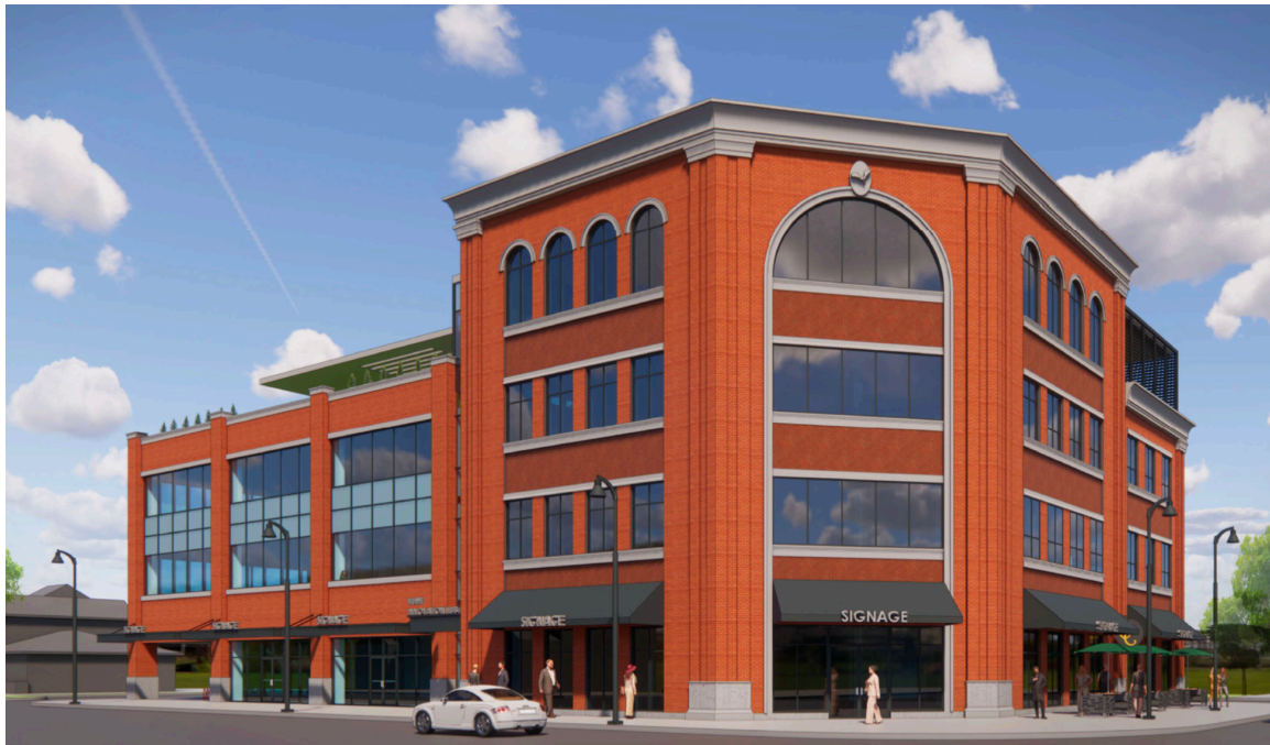
Figure 5 – Original Building Façade
