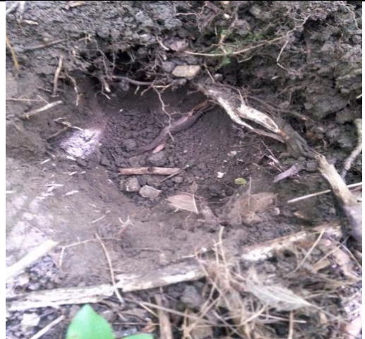
IMAGE 14 VIEW OF COMPLETED TEST PIT
