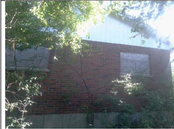
IMAGE 3 VIEW OF STRUCTURE
