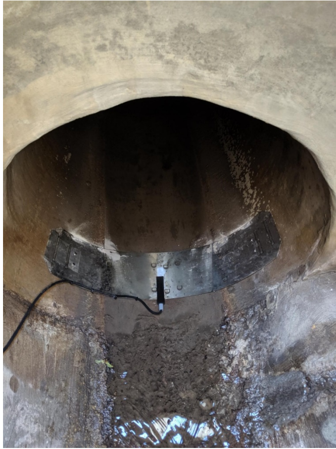
Figure A4- 6 SM_256 Monitor Installation
