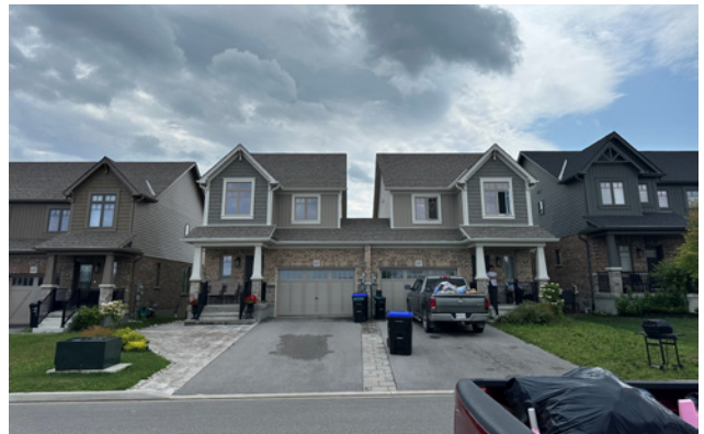
Block 266 in Phase 2 showing three sets of semi-detached unit blocks with varying facade materials to create visual interest
