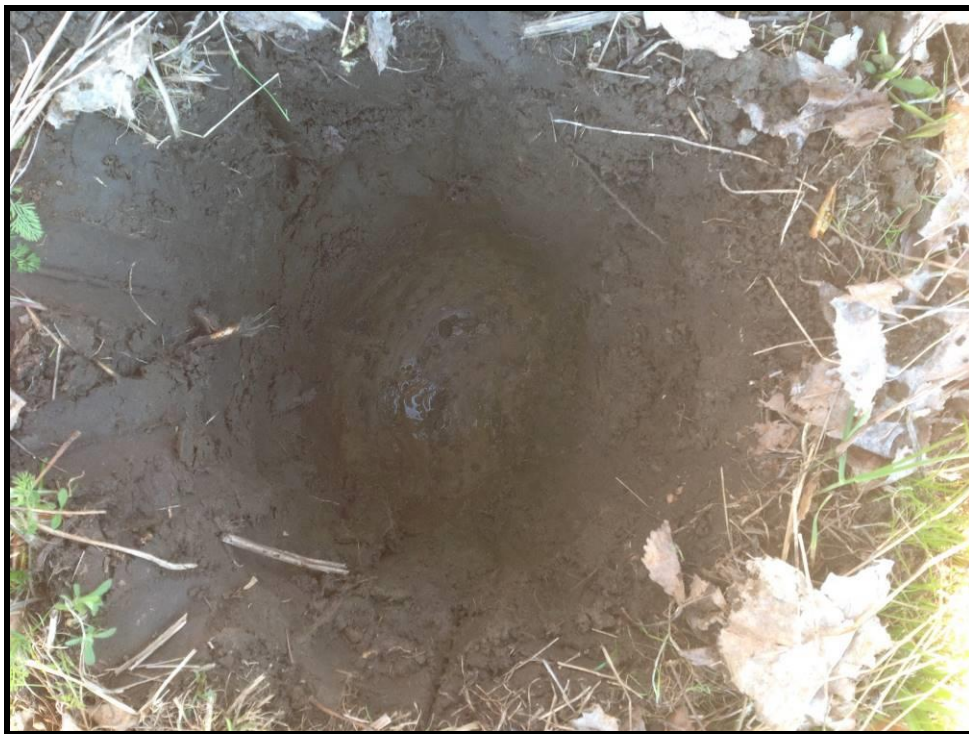
Image 13: Typical Test Pit (Photo Taken on May 1, 2015; Facing North)
