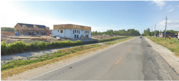
Figure 1.2 : Looking north along High Street towards the partially built, prior phases of the Summitview development
