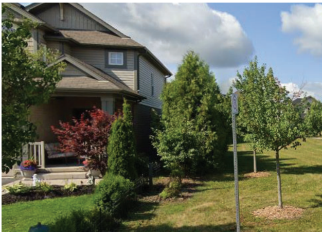
Figure 4.7 : Examples of residences adjacent to open spaces showing side facades with material enhancements
