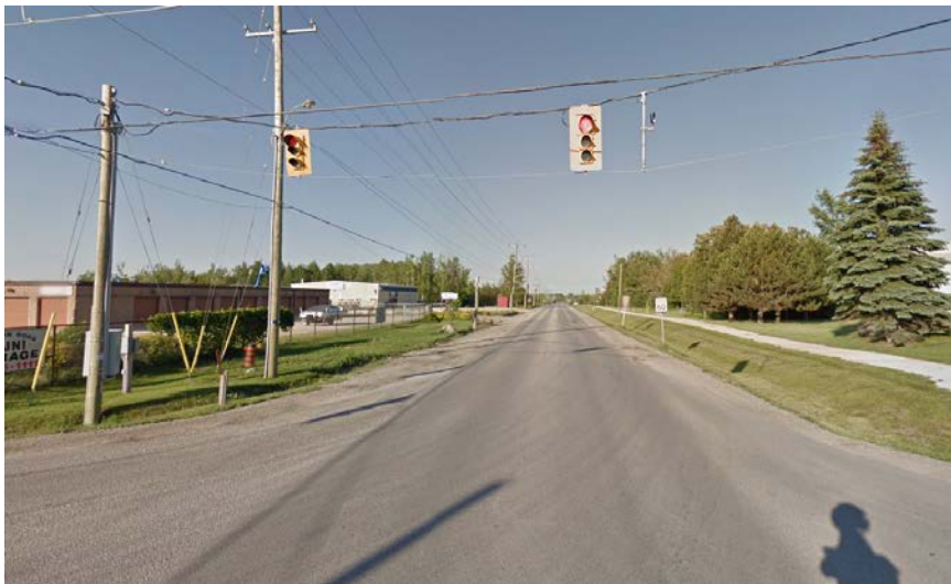
Looking east along Mountain Road from Tenth Line
