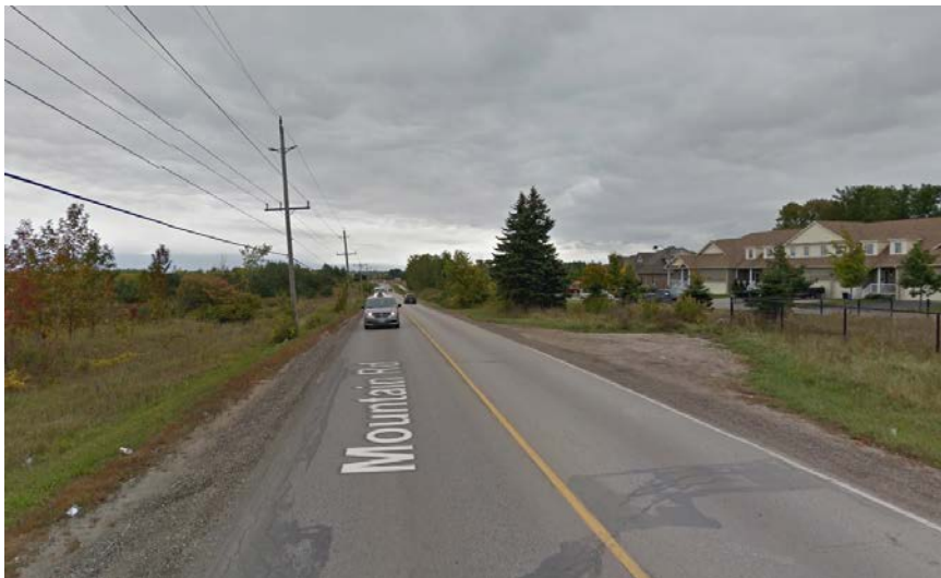
Looking east along Mountain Road from Site Access 2
