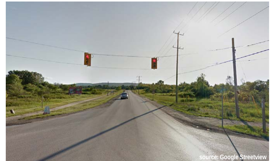
Looking west along Mountain Road from Tenth Line
