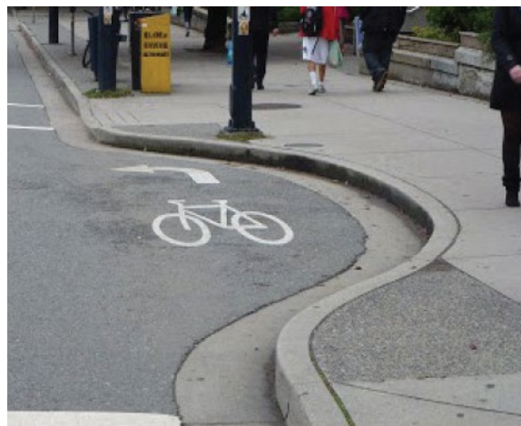
FIGURE 3.2: BIKE JUG HANDLE AT A T-INTERSECTION (Source: OTM Book 18, Figure 4.52, p. 85)
