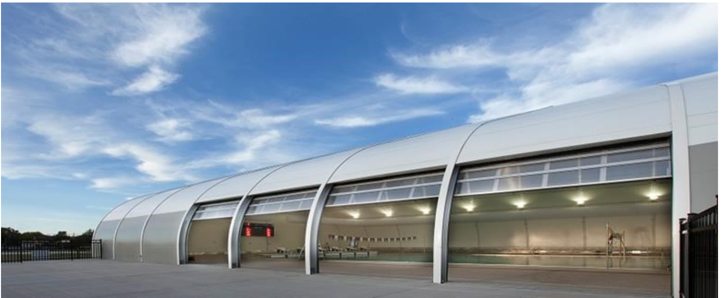
CENTENNIAL AQUATIC CENTRE
