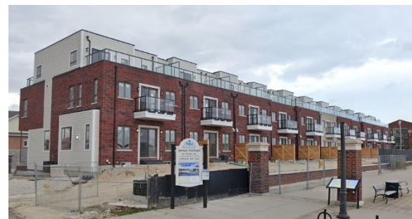
Existing Side Launch Townhomes
