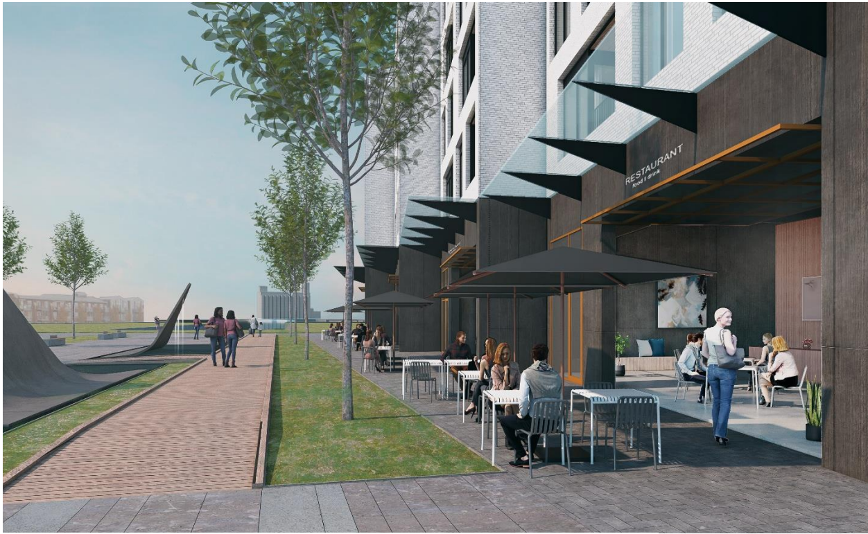
North view towards to water of the proposed retail adjacent to the future town Piazza
