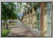
Example of weather protection provided by a canopy structure that allows sunlight through, and is designed to fit with, the architectural style of the building.
