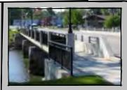
This large multiple lane bridge is designed with a dedicated pedestrian walkway that is physically separated from traffic as per the UDM requirements.
