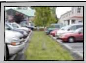
Example of a stormwater management bioswale used in a parking lot.
