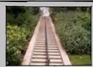
Bike ramps installed along a stairway to assist cyclists.
