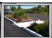
Pictured is an example of a walkway design that allows stormwater to enter a planter area as part of a Low Impact Development stormwater management system.
