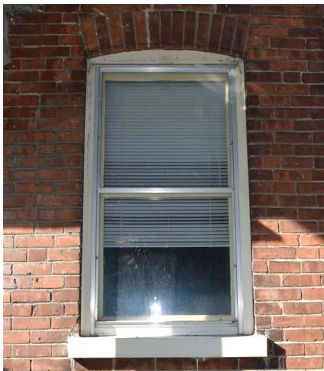
Figure 18: Segmental arch window.
