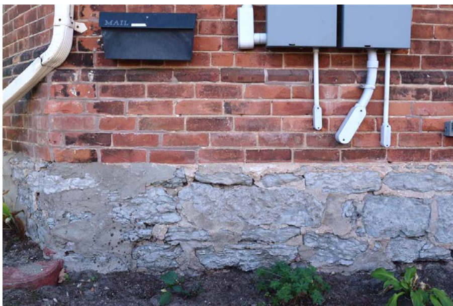
Figure 19: Coursed rubble foundation and brick water table.
