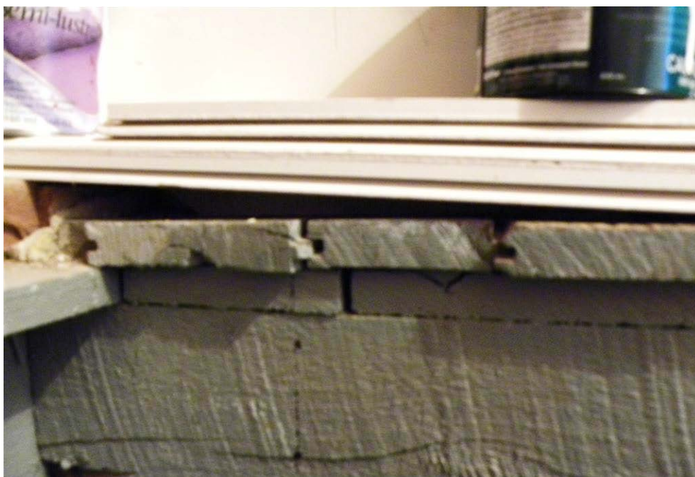
Figure 33: Tongue-and-groove floorboards visible on the basement staircase.
