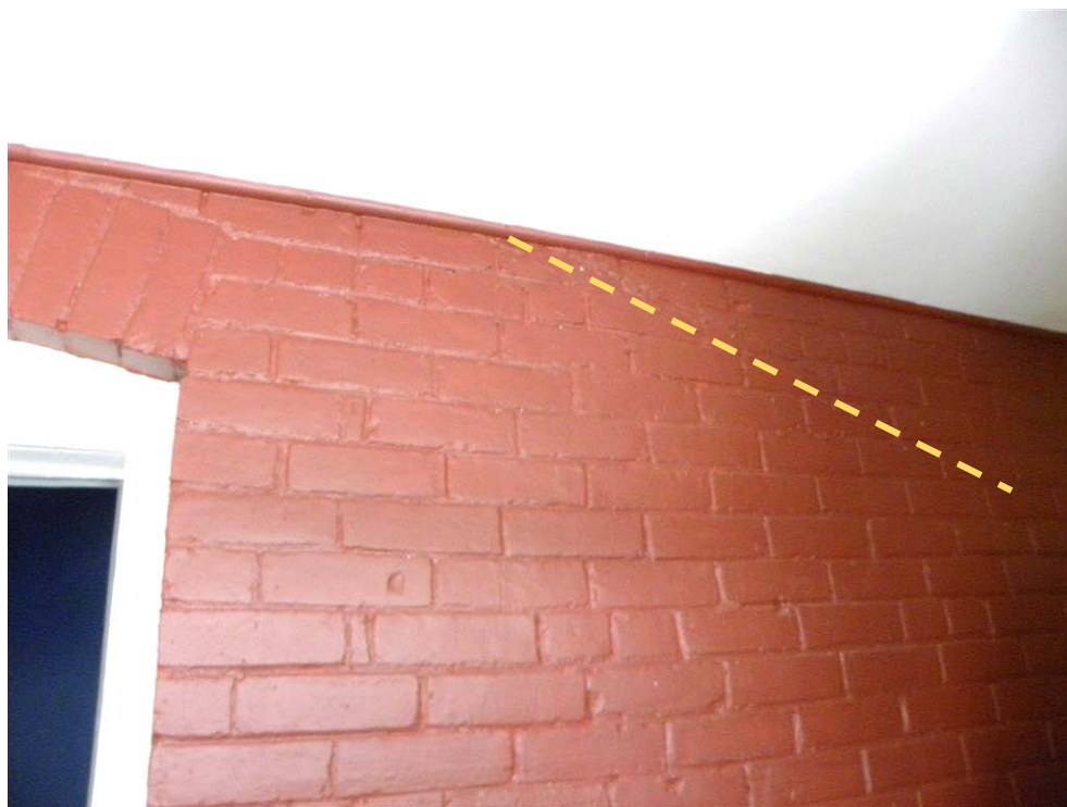
Figure 28: Roof scar within the current wood mud room, highlighted with a yellow dashed line.
