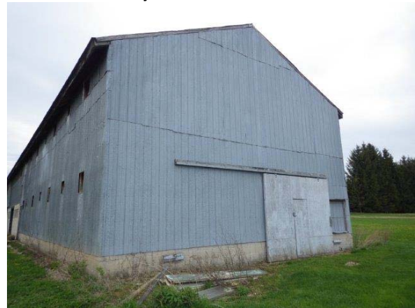
10. Barn structure located on 7914 Poplar Sideroad (Phase One adjoining property).
