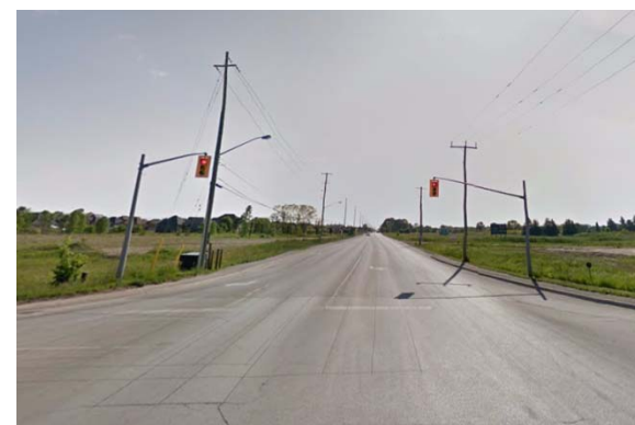
Looking east along Poplar Sideroad from Hurontario Street
