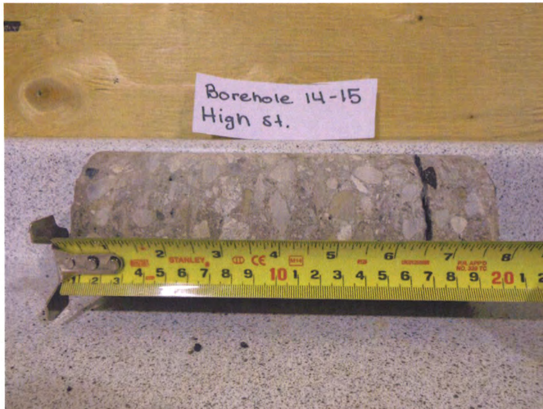
Figure # 6: Borehole 14-15 – High St., Collingwood, Ontario
